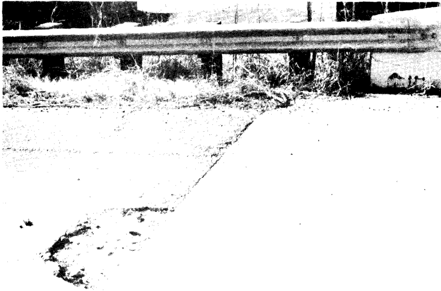
Parish Road Overpass - I-20, Station 238+00 No sign of embankment distress. However, a pavement failure is to the left.
