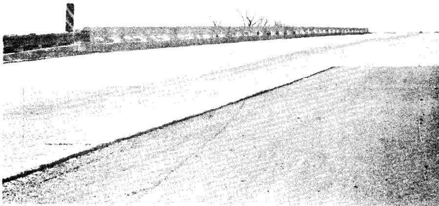
I-20 Overpass - M.P.R.R. and Walnut Bayou Station 904+00 Looking west on the eastbound roadway. Structure is over M.P.R.R.
