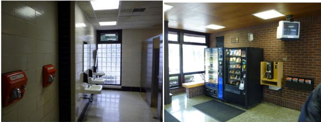
Figure3: Lobby and Restroom Lights on Near Windows Despite Ample Daylight
