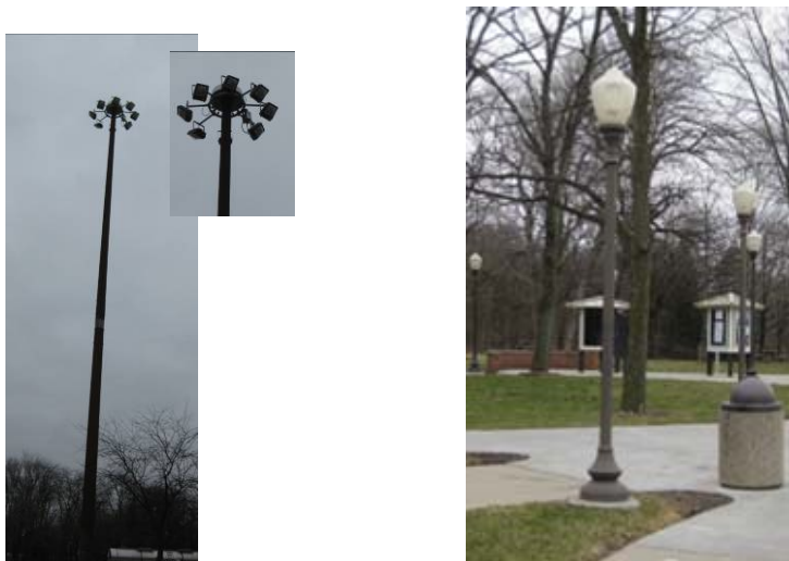
Figure 27. Lighting tower and exterior lighting poles of Funks Grove rest area.
