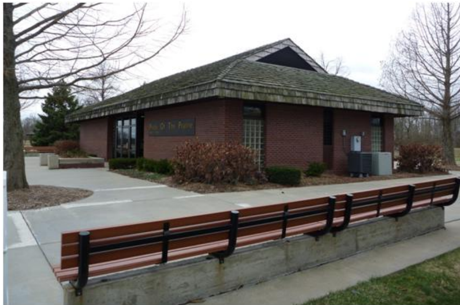
Figure 2: Exterior View of the Eastbound Rest Area
