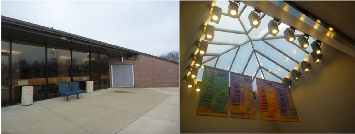
Figure 2: Rear Entry Vending Area, Lobby Lighting Shining Down and Up into Skylight
