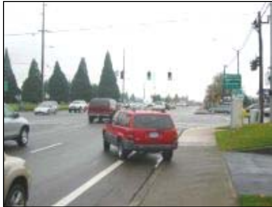
Figure 5.7: Driveways near intersection, driveway spacing
