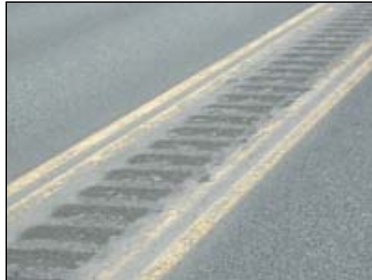
Figure 3.11: Centerline rumble strips
