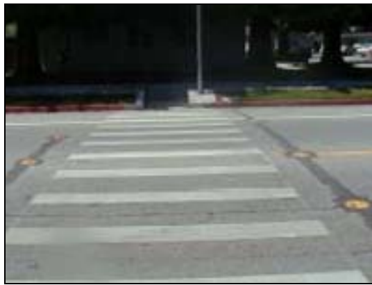
Figure 5.27: Flashing lights in crosswalk
