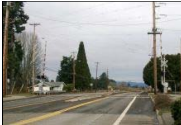
Figure 5.30: Active warning device
