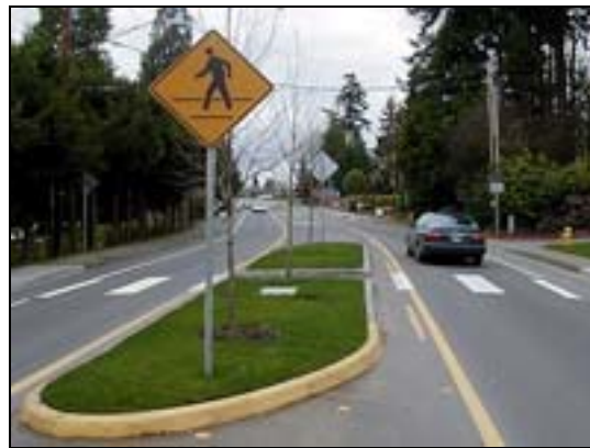
Figure 5.29: Marked mid-block crosswalk
