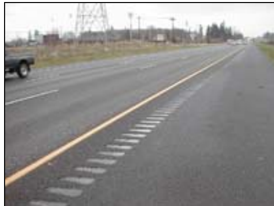
Figure 3.13: Shoulder Rumble Strips
