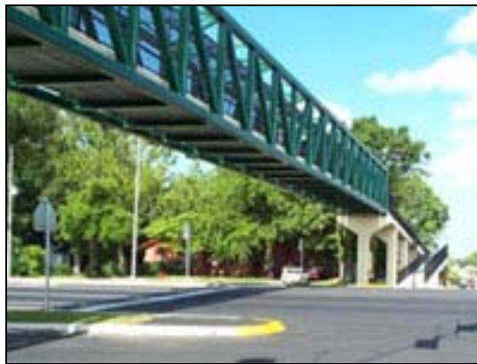
Figure 5.26: Pedestrian grade separation
