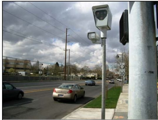
Figure 3.16: Automated enforcement of red light violations
