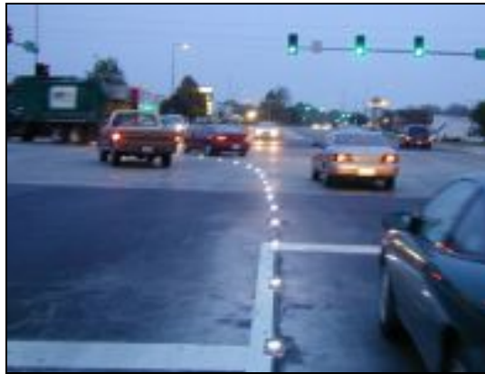
Figure 5.11: Turning guide lines for multiple left-turn lanes
