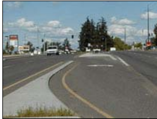
Figure 3.2: Left-turn bay, unsignalized intersection
