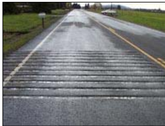
Figure 5.10: Transverse rumble strip in advance of stop controlled intersection
