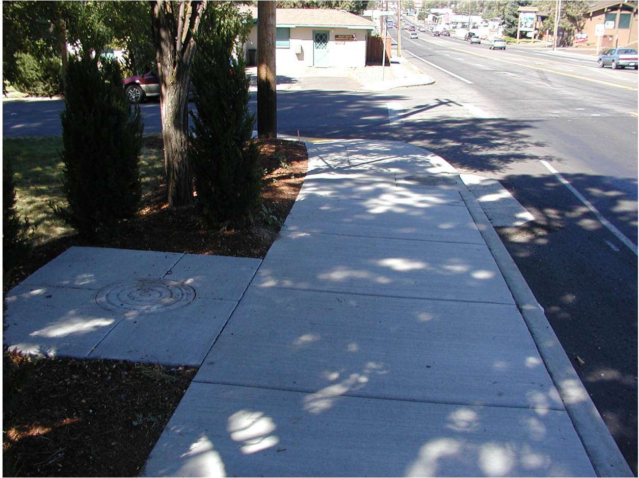
Drain straight to dry well at west end of Highway 20 project in Bend, Oregon beside Pilot Butte.
