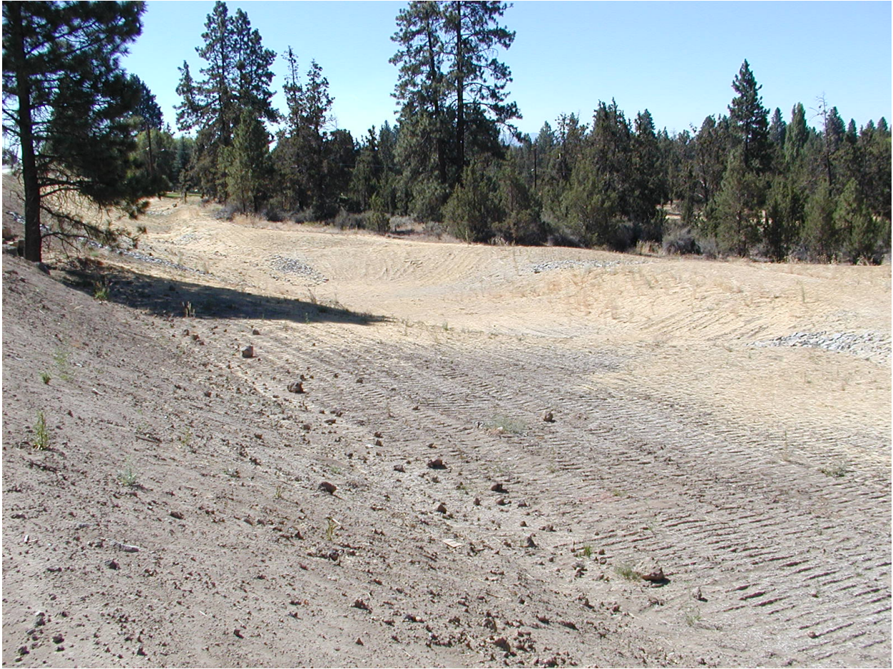
Detention ponds for middle section of Highway 20 project in Bend, Oregon beside Pilot Butte.
