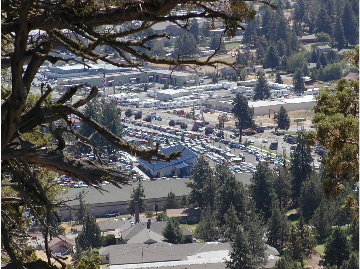
Eastern end of Highway 20 Project in Bend, Oregon beside Pilot Butte. Large storm water detention and storage pipe is being laid in the center of the roadway along with oil-water separators and dry wells.
