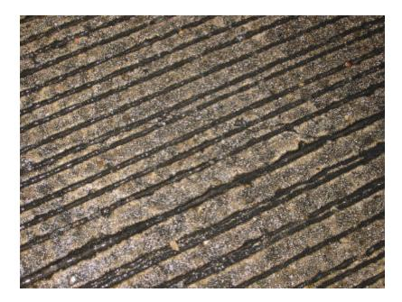
Figure 17 Photograph of cracks in concrete slabs В В В В е Ň е е е nt Span(1) Span 3 Span(2) ņt short span nt pt 3 Joint Joint Visible Cracks To Baton Rouge Plan View
