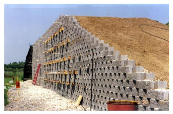
Figure 21 View of the pullout boxes at the vertical facing of the wall
