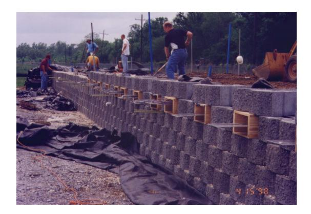
Figure 23 View of the first layer of pullout boxes during construction
