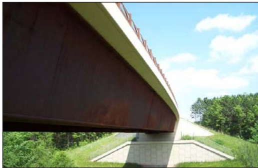
East side of bridge, looking north
