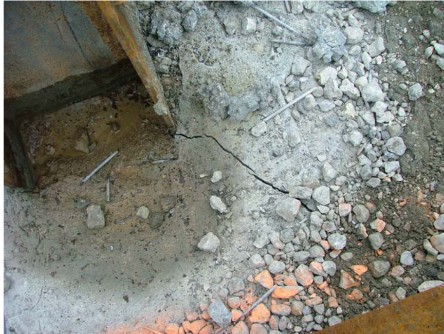
Figure 47: Cracking at 556 kN-667 kN (125,000 lb-150,000 lb)
