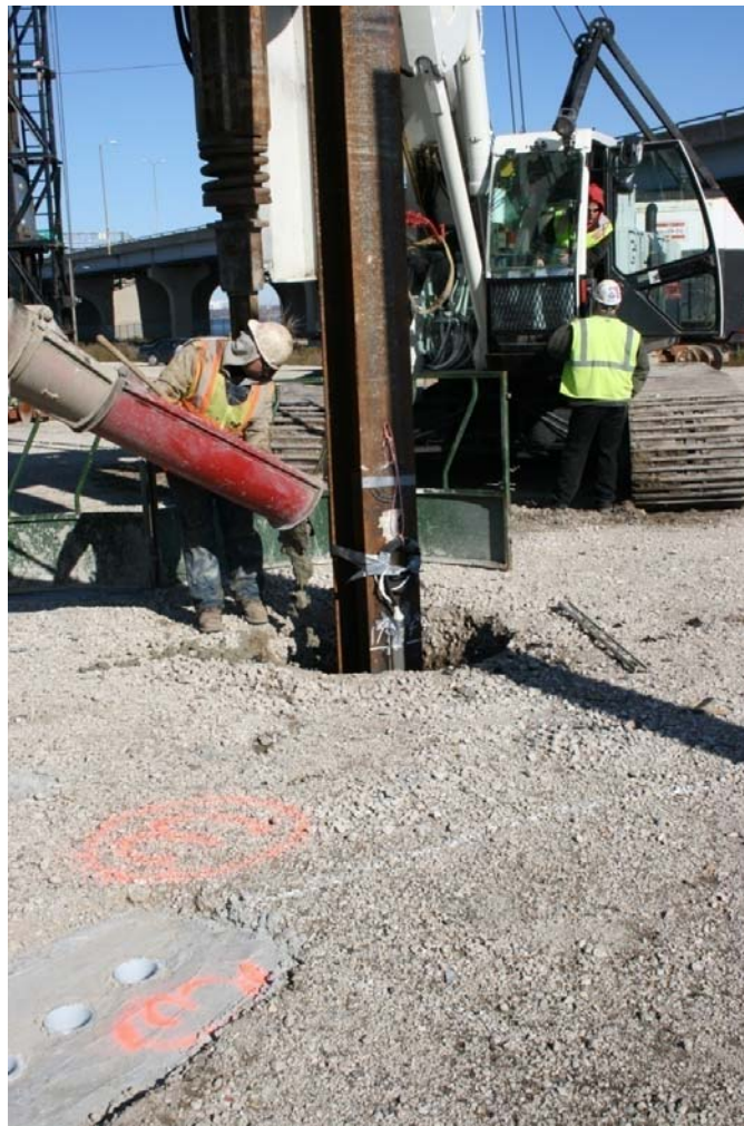
Figure 39: Installation of the Pile with Concrete Pier
