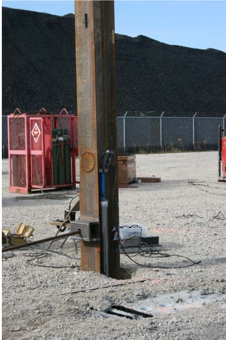
Figure 30: Loading Mechanism for the Pile with Steel Plate
