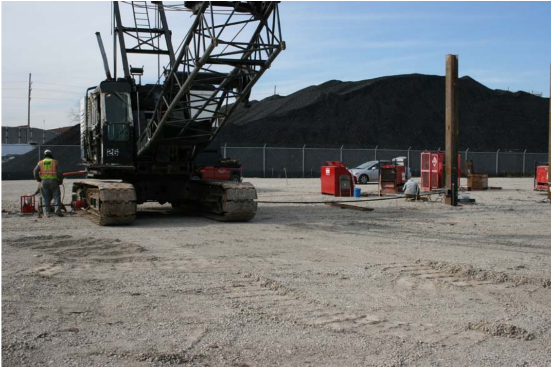
Figure 31: Loading Mechanism for the Pile with Steel Plate
