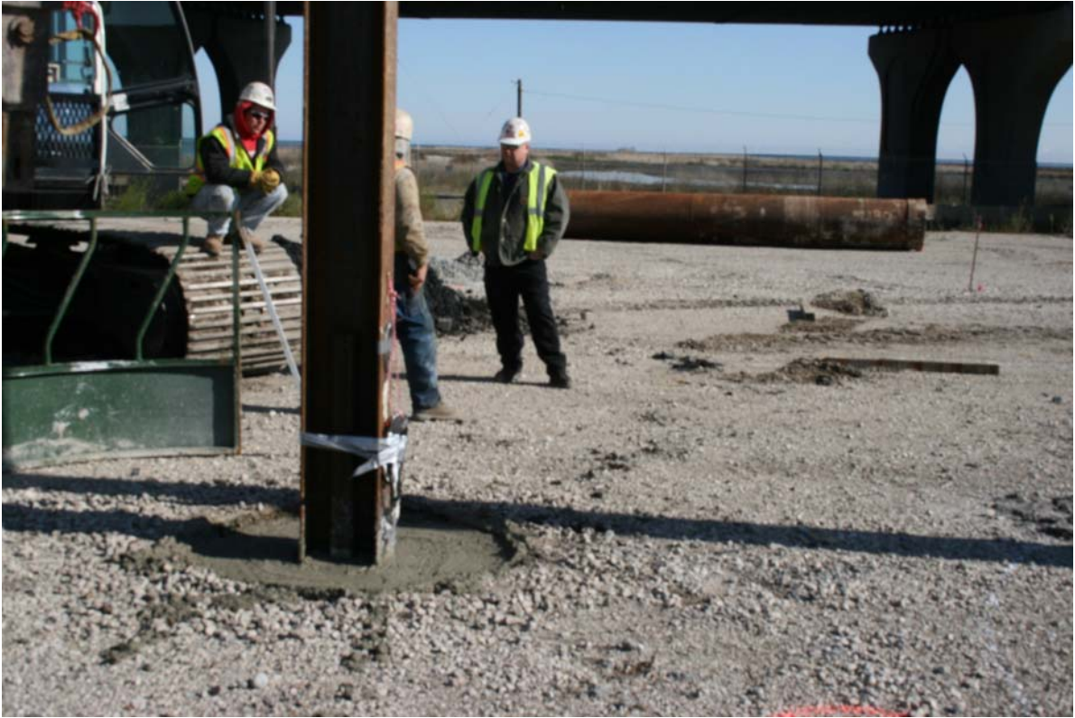
Figure 40: Installation of the Pile with Concrete Pier
