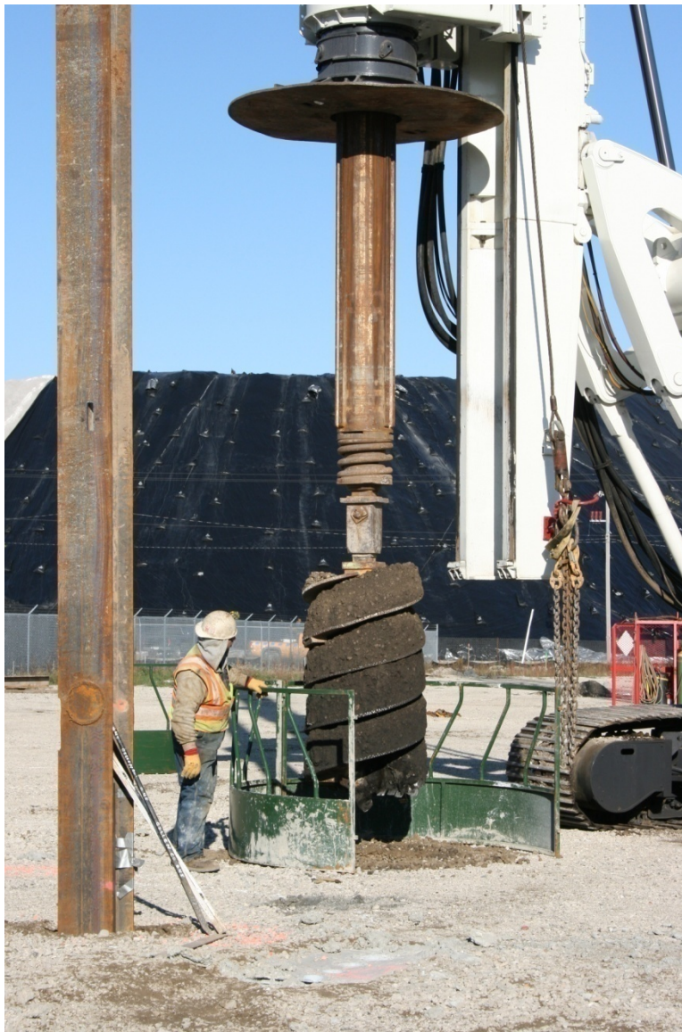
Figure 37: Installation of the Pile with Concrete Pier
