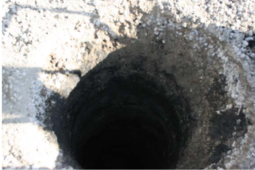
Figure 38: Installation of the Pile with Concrete Pier
