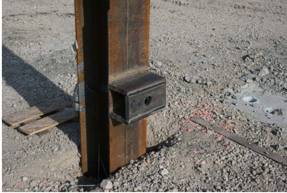
Figure 29: Loading Mechanism for the Pile with Steel Plate
