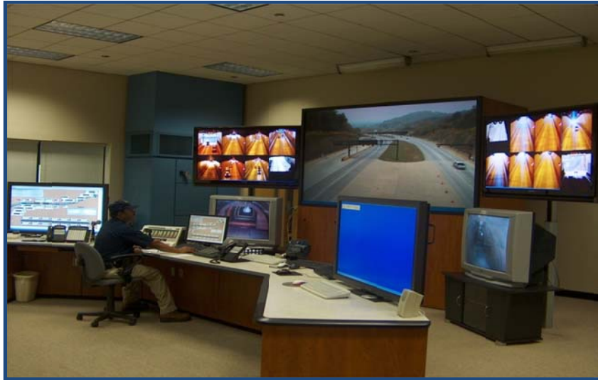
Figure 5. CGT Control Room Circa 2007
