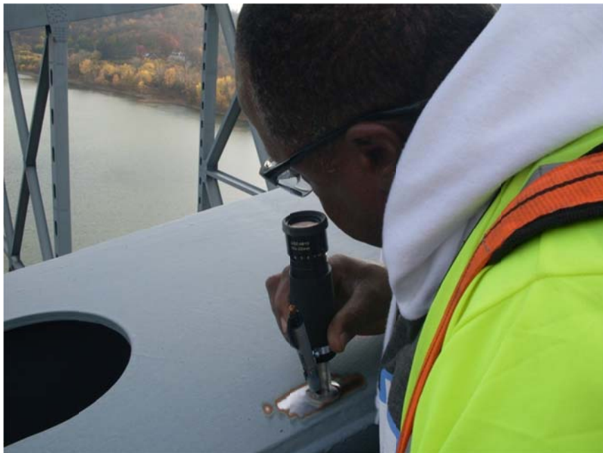
Figure 15. NDE Technician Measuring Telebrineller Mark Diameter on an Upper Chord Member of the I-275 Westbound Bridge.
