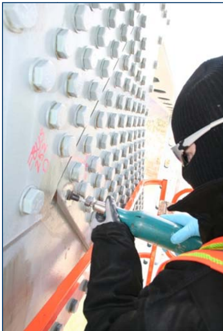
Figure 22. HTT NDE Supervisor Performing Ultrasonic Shear Wave Inspections on a 1/2" Splice Plate on the Downstream Truss of the Westbound Bridge.
