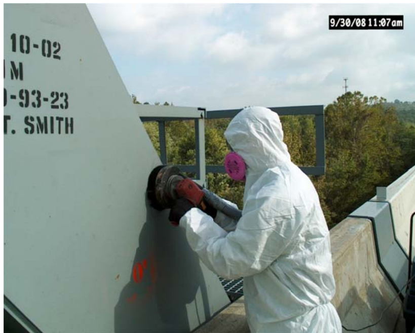
Figure 18. Intech Worker In-training to Remove Leaded Paint for Test Patches.
