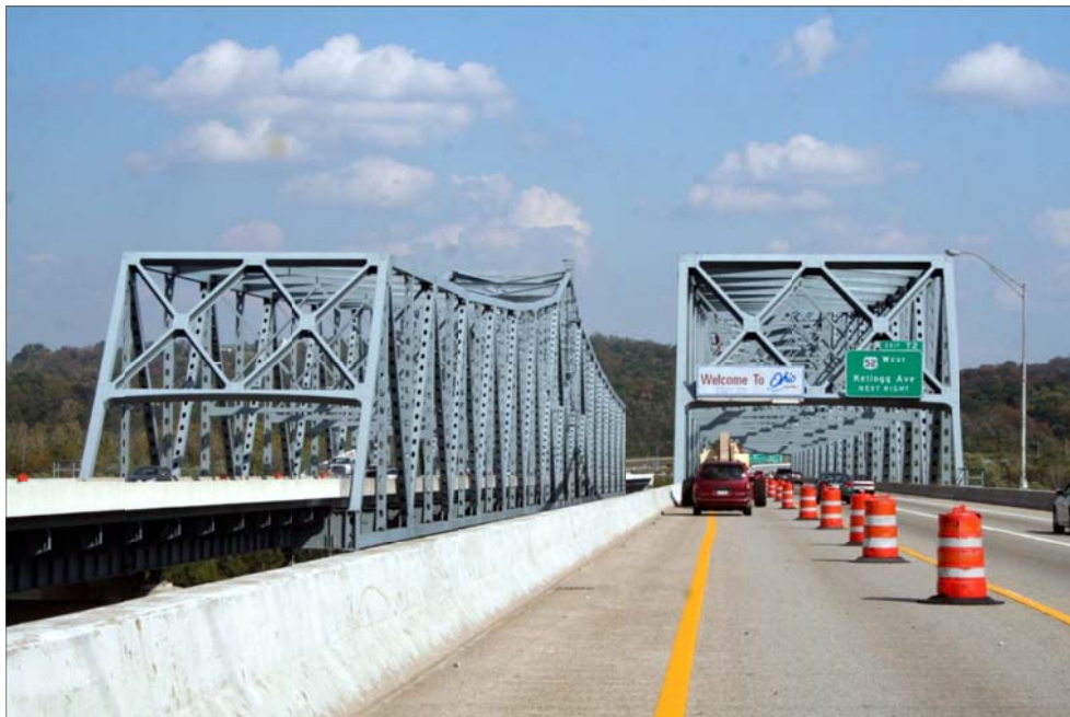
Figure 17. Lane Closure Set-up on the Eastbound Bridge (10/13/08).
