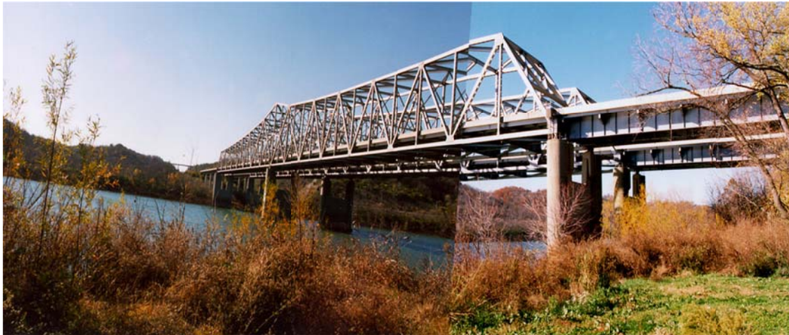
Figure 1. I-275 Combs-Hehl Twin Bridges over the Ohio River (Courtesy J. Mecklenborg).
