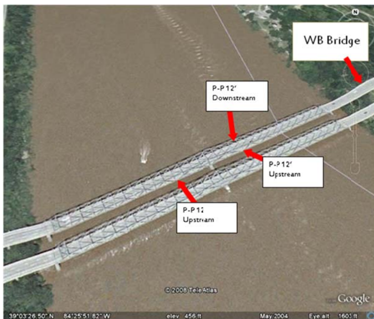
Figure 3. I-275 Combs-Hehl Twin Bridges Showing Locations of Cracked Splice Plates on Westbound Bridge.
