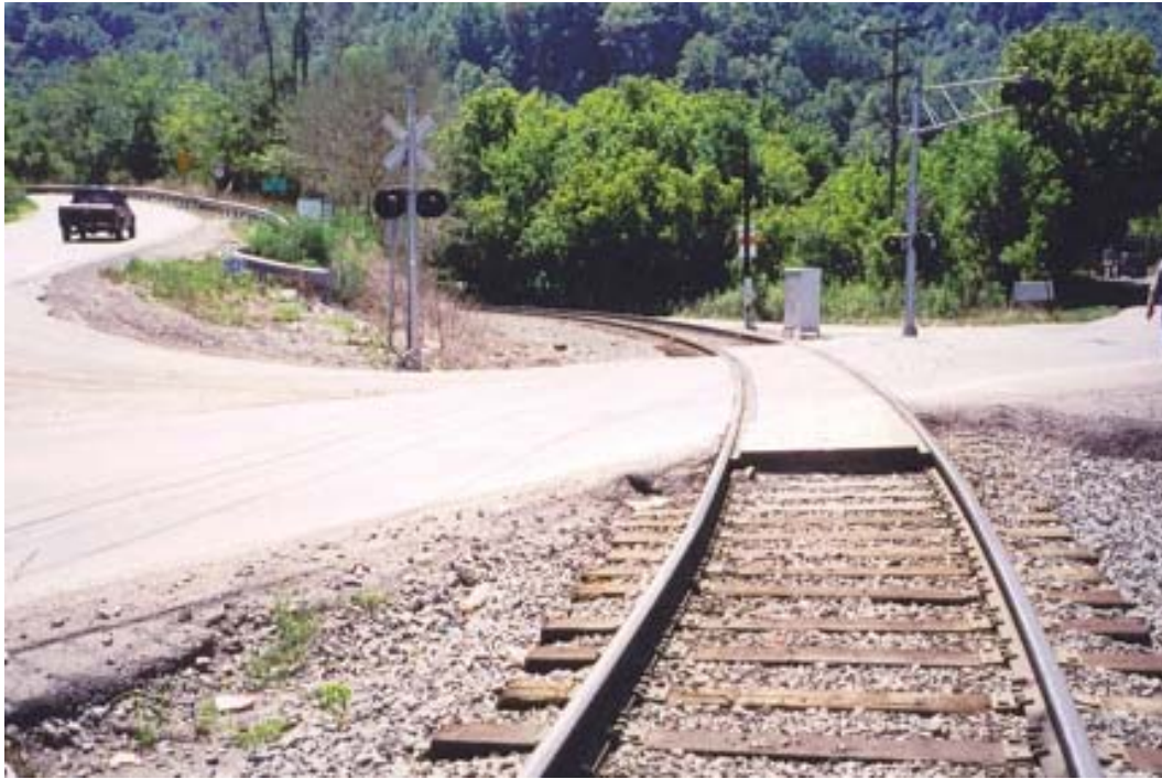
Figure 2.4.2a. Rehabilitated Crossing in Lackey, Kentucky
