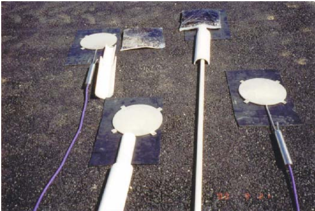
Figure 2.4. Pressure Cell Installation
