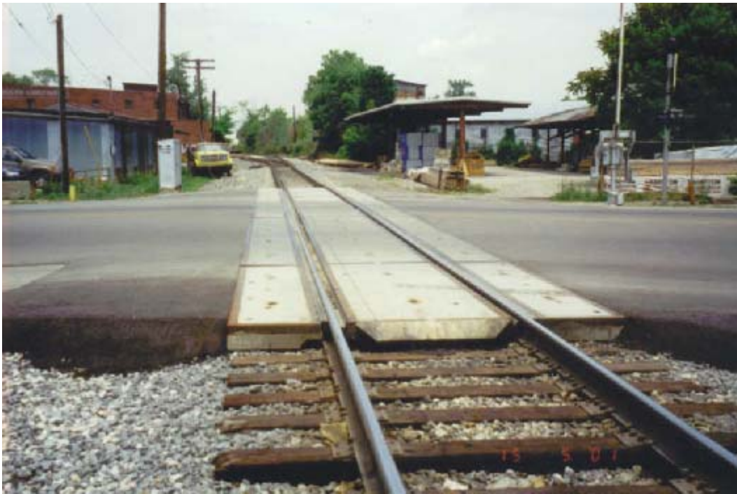
Figure 2.4.1a. Rehabilitated Crossing in Richmond, Kentucky
