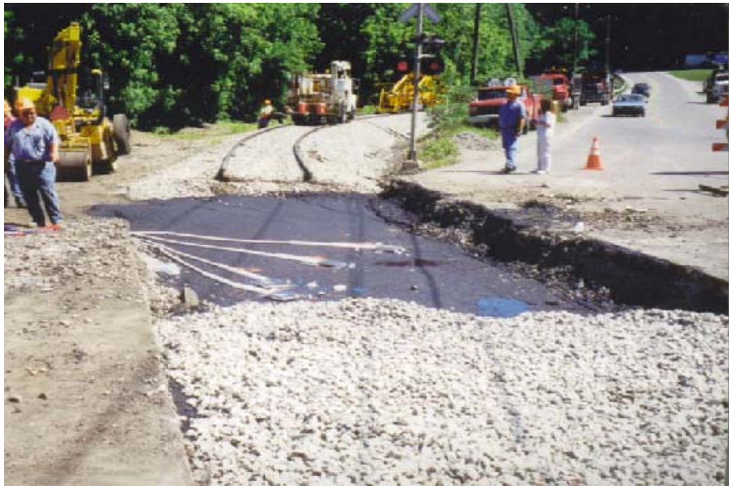
Figure 2.4.2b. Pressure Cells Placed on the Asphalt Layer
