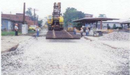
Positioning wood tie panel
