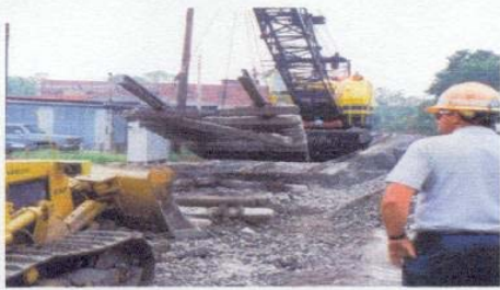
Lifting out old Panel
