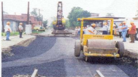
Compacting asphalt
