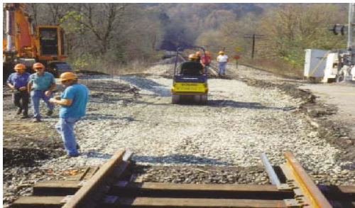
Compacting ballast 11:20
