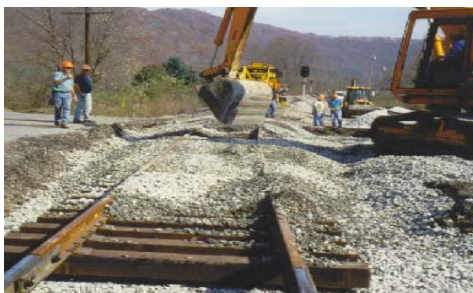
Compacting hand-spread approaches
