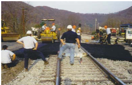
Spreading cribbing rock 11:30
