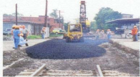
Compacting placement of asphalt
