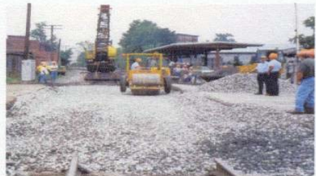
Compacting ballast
