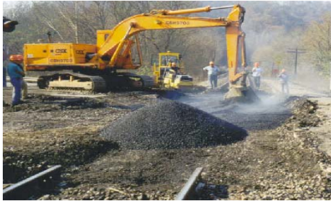
Spreading asphalt
