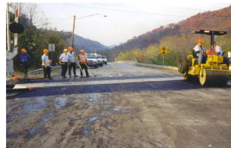
Finished compacting asphalt approaches 16:50
