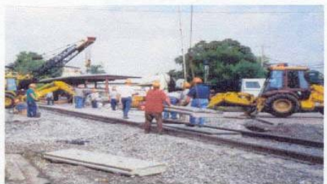
Placing concrete surface
