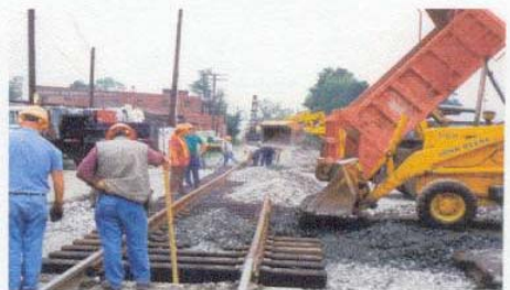
Dumping cribbing rock
