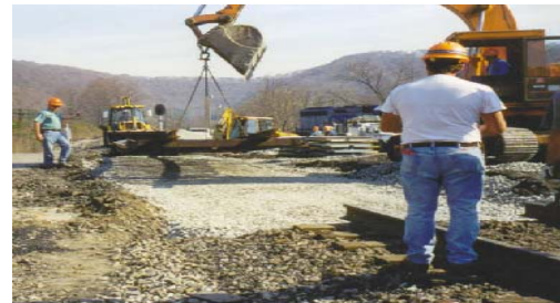
Positioning new panel
