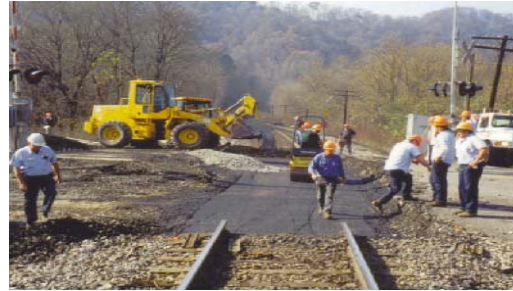
Compacting asphalt and dumping ballast
