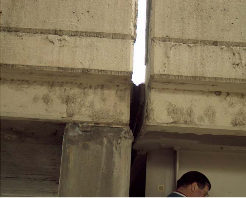
Figure 35. Closed deck joint in good condition (April 2009).
