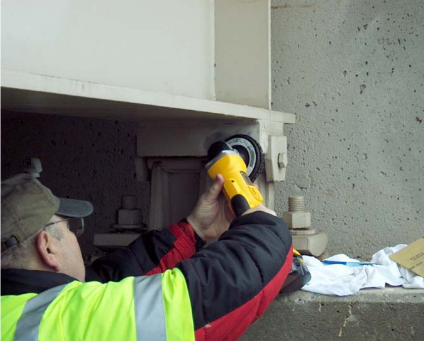
Figure 31. Removing paint to conduct soluble salt test at steel substrate (April 2009).
