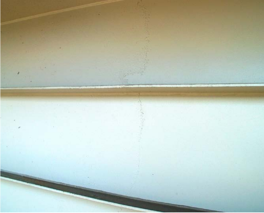
Figure 37. Ragged edge between existing paint on right and new paint on left (April 2009).
