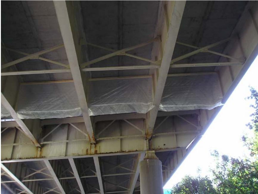
Figure 3. Bulkheads installed adjacent to a joint prior to cleaning and painting.
