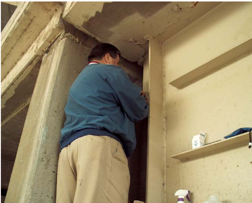
Figure 30. Conducting soluble salt test on steel on deck joint (April 2009).
