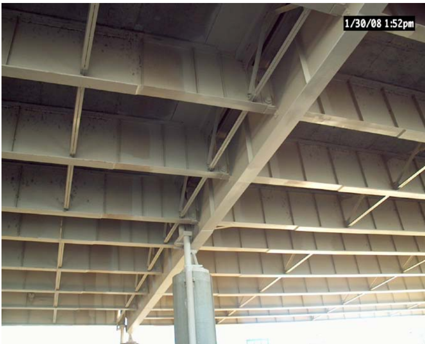
Figure 26. Overall view of zone painted area in good condition (January 2008)
