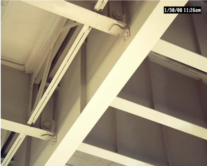
Figure 25. Zone painted floor beam and girders in good condition (January 2008).
