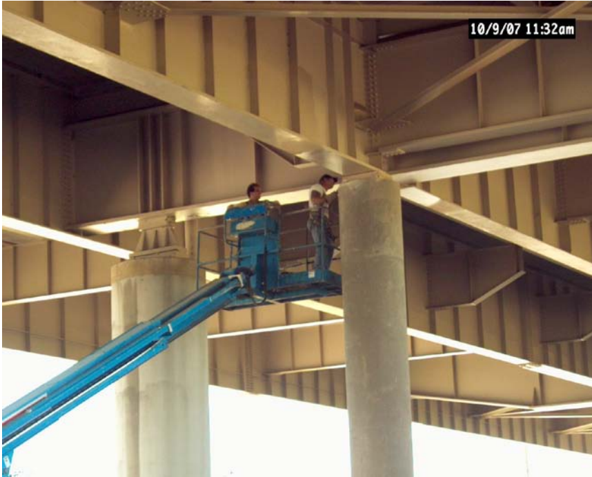
Figure 21. Inspector examining completed coating at joint.
