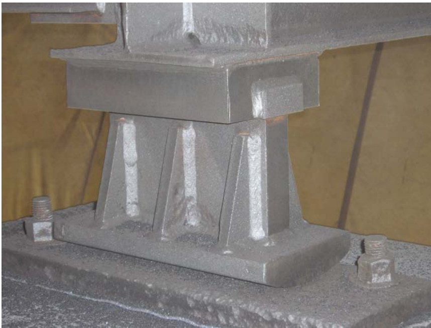
Figure 12. Properly blast-cleaned rocker at abutment ready for painting.
