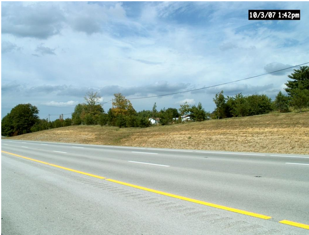
Figure 2 Pilot Program Site at mile marker 92 on I 64 Westbound near Lexington, KY
