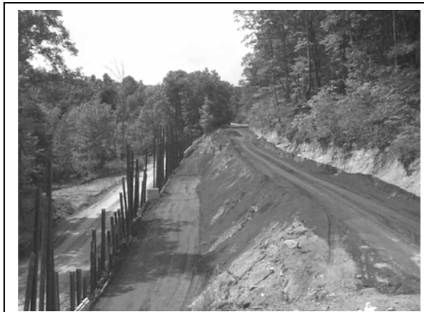
Figure 1. Bottom ash from a coal-fired electric power plant used in a landslide correction in McCreary County, Kentucky.
