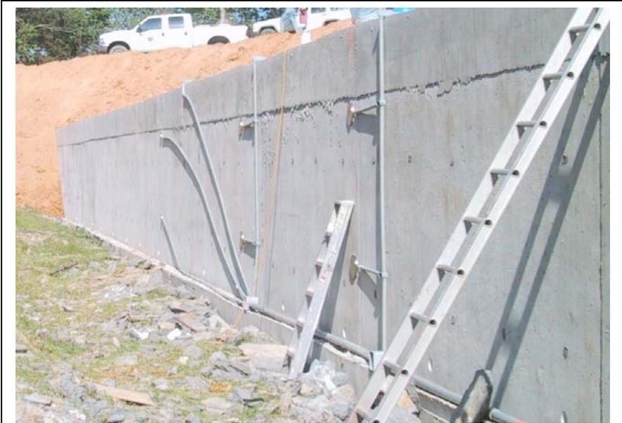
Figure 20. Wires are protected and guided to culvert bottom.
