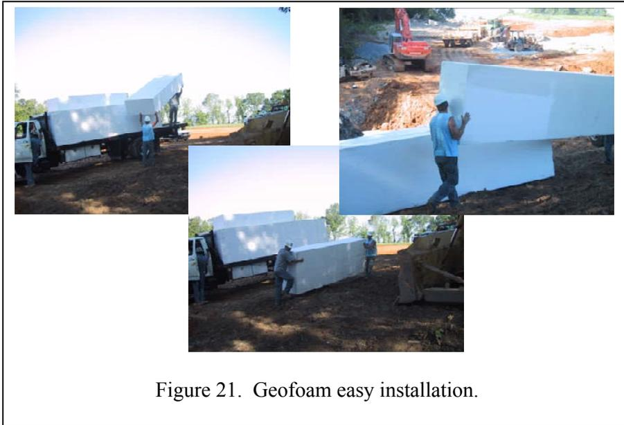
Figure 21. Geofoam easy installation.
