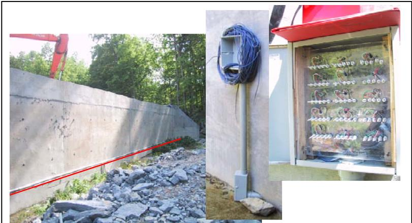
Figure 16. Grouped wires and reading station
