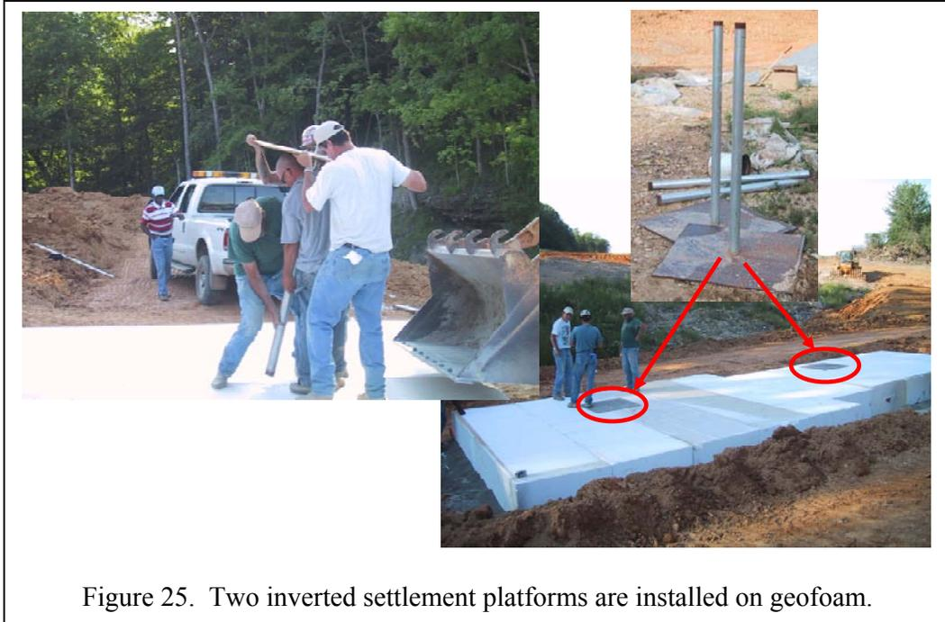
Figure 25. Two inverted settlement platforms are installed on geofoam.
