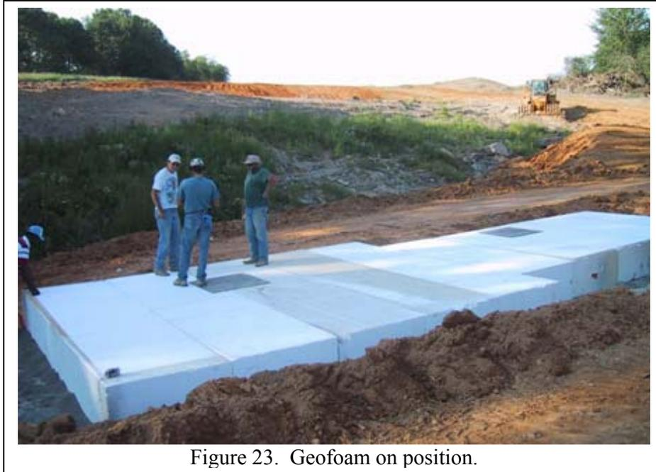
Figure 23. Geofoam on position.
