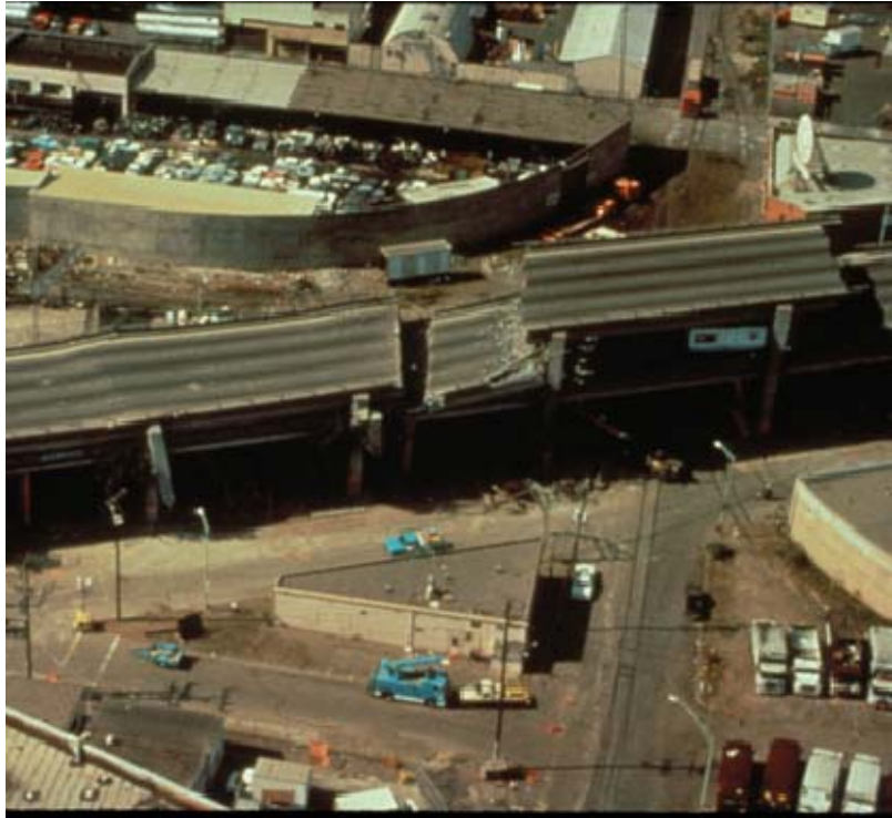
Figure 1-4. I-80 damage during the 1989 Loma Prieta earthquake.
