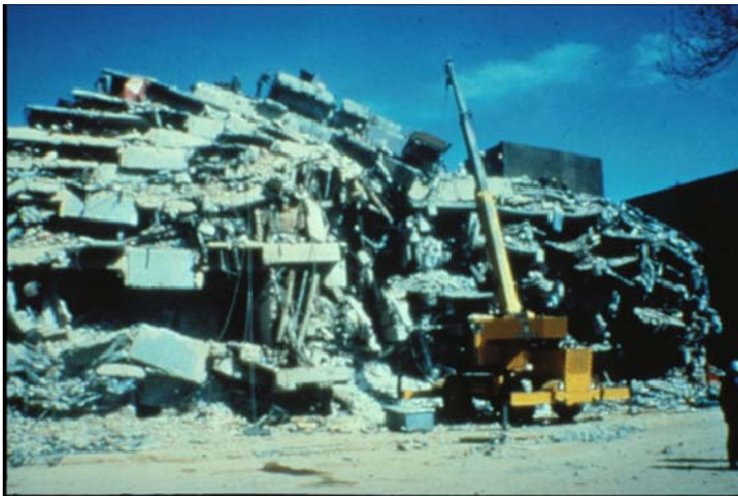
Figure 1-5. Complete destruction of a building caused by amplified ground motion in Mexico City during the 1985 Mexico earthquake.
