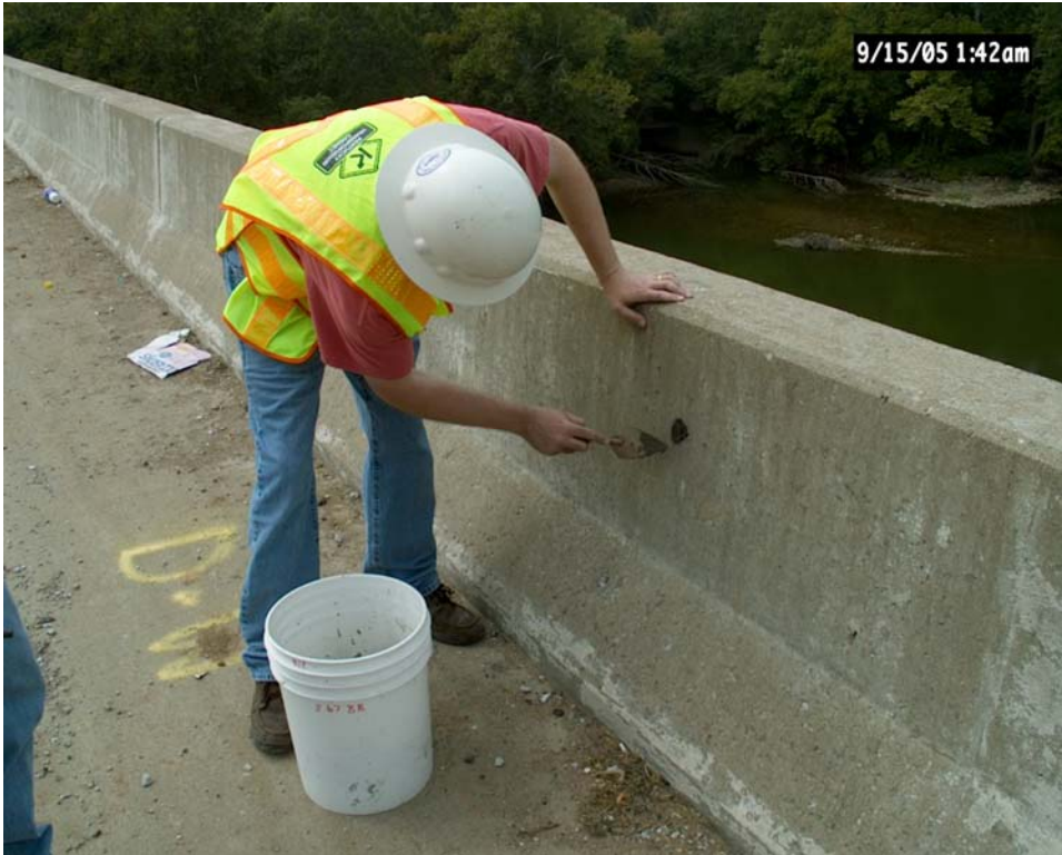
Figure 15. Patching the drilled holes with Tamms Speedcrete Redline
