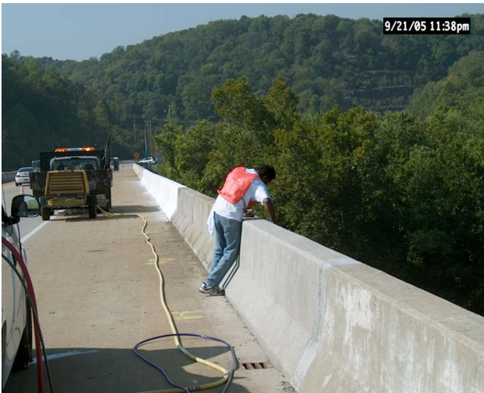
Figure 18.Rolling 12" patch of coating system on the back of barrier wall
