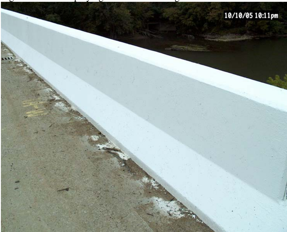
Figure 20. Finished spraying of a concrete coating on the barrier wall
