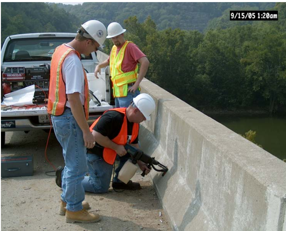
Figure 14. Drilling barrier wall for taking concrete samples for baseline chloride data
