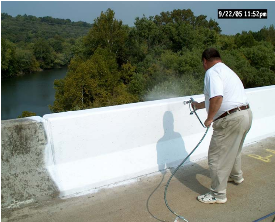
Figure 19. Airless spraying of concrete coatings on the barrier wall
