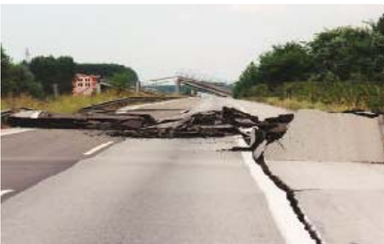
Figure 22 Severe Damage. Damage to the roadway due to fault rupture. (3)
