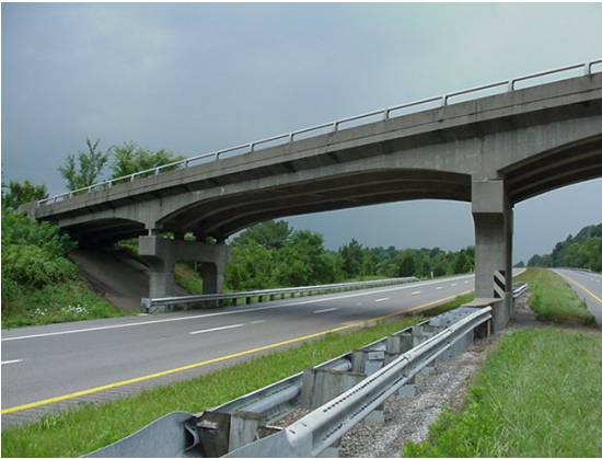
Figure 9 "Haunched" Concrete Girder Bridge (25)
