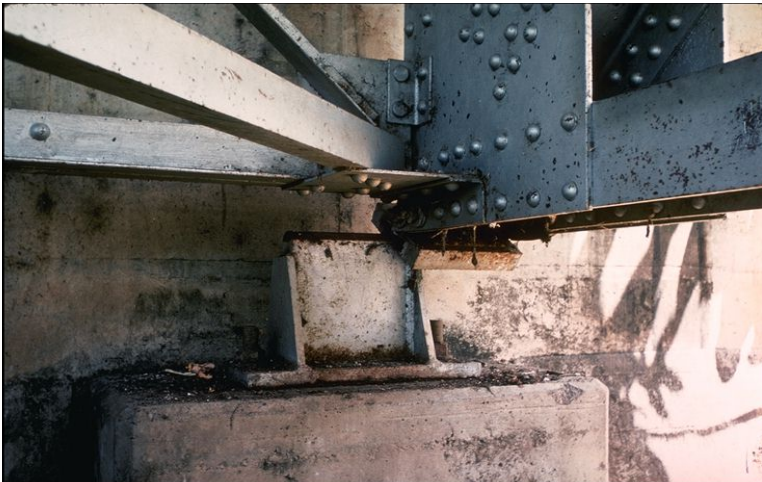
Figure 57 Severe Damage. Displacement of the steel girder off the bearing support. (1)
