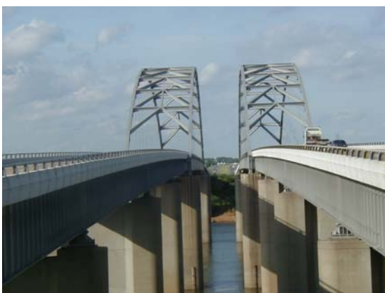
Figure 17 Plate Girder Bridge with Steel Arch (25)
