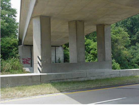
Figure 7 Cast-in-Place Box Girder Bridge (25)
