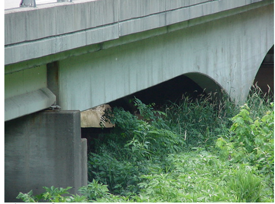
Figure 8 "Haunched" Concrete Girder Bridge (25)
