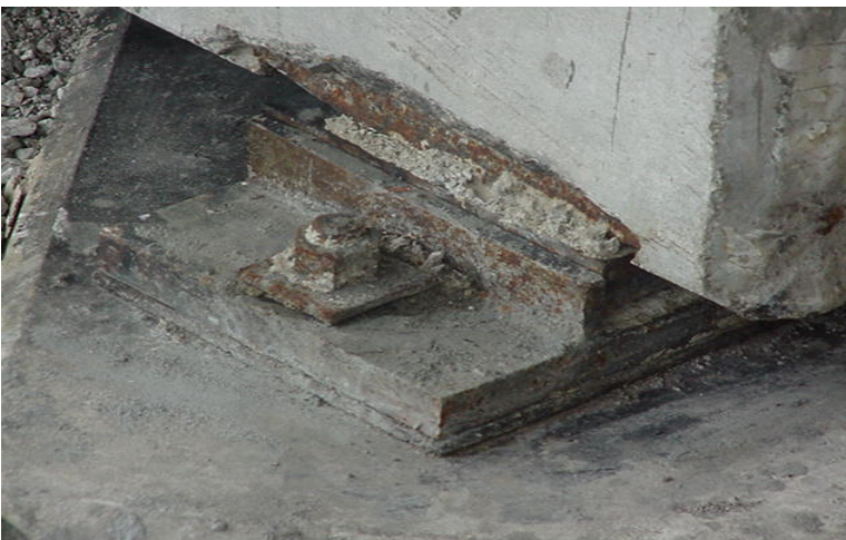
Figure 24 An already corroded “slider” type bearing assembly is susceptible to transverse shearing forces induced by seismic demands and may pose a threat of collapse if the displacements become excessive once sheared. (25)
