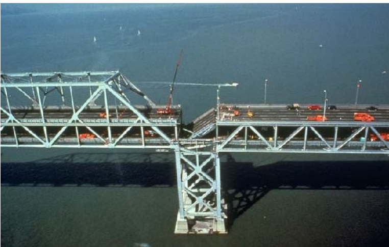
Figure 58 Total Failure. Unseating at the expansion joint. (1)
