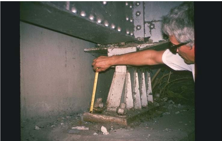
Figure 55 Moderate Damage. Crushed bearing assembly. Also note the slightly elongated bolts. (1)
