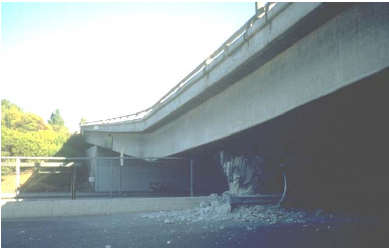
Figure 28 Severe Damage. Excessive damage to the superstructure and the substructure has caused partial collapse to the bridge, rendering it unsafe for traffic. (1)
