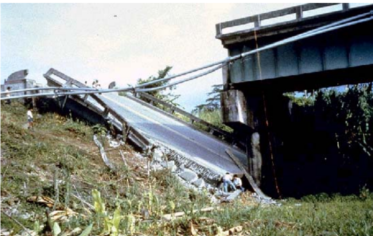
Figure 36 Total Failure. Collapse of the simply supported span due to anchor bolt failure and spalling of the concrete cover. (11)
