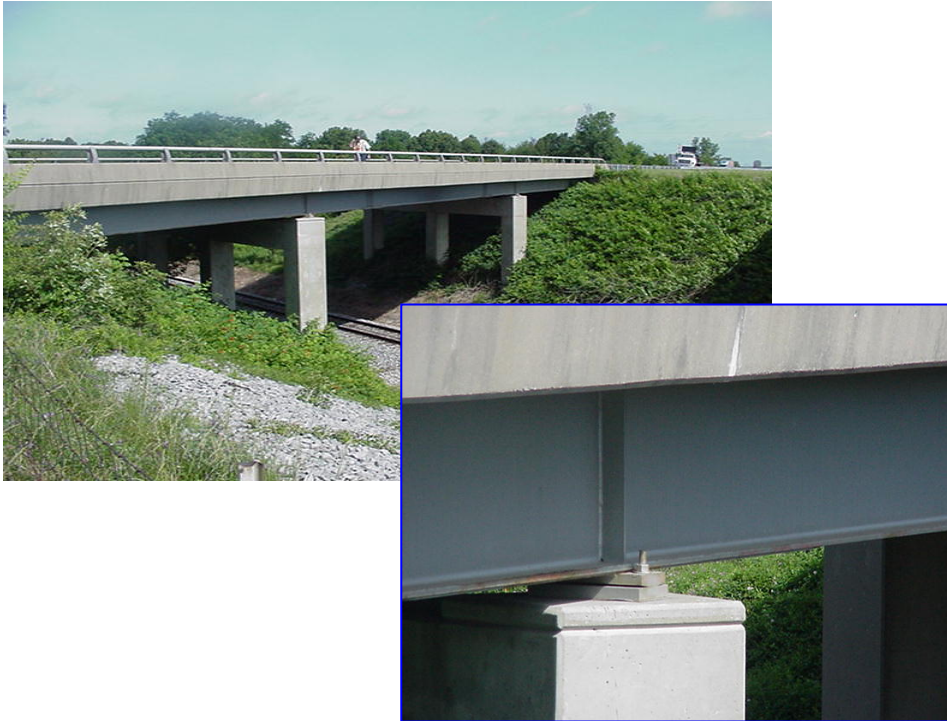
Figure 31 Continuous steel plate girder bridge. (25)
