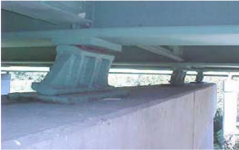
Figure 50 No Damage. Movement of the rocker bearing due to thermal loads. (13)
