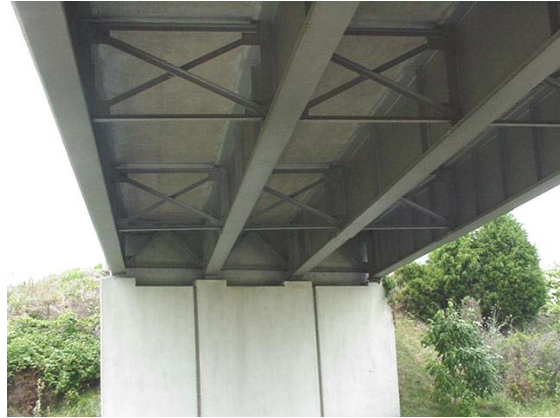
Figure 14 Welded Plate Girder Bridge (25)
