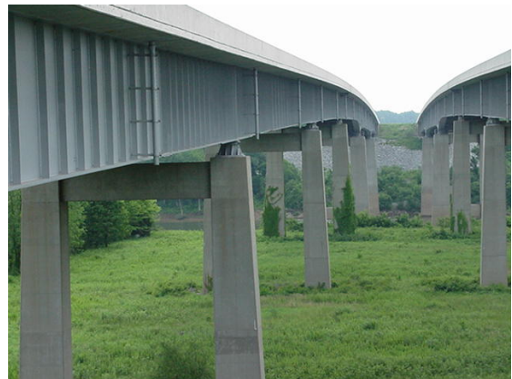
Figure 12 Continuous Welded Plate Girder Bridge (25)
