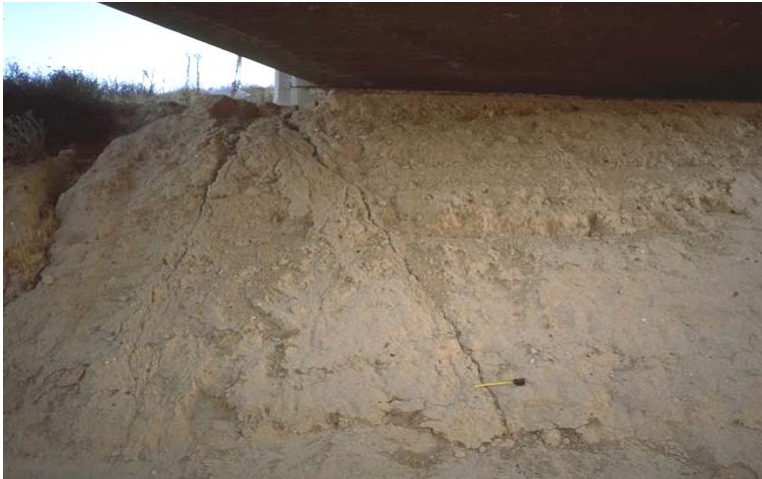
Figure 18 Minor damage. Ground crack extending diagonally down slope under the abutment. (1)
