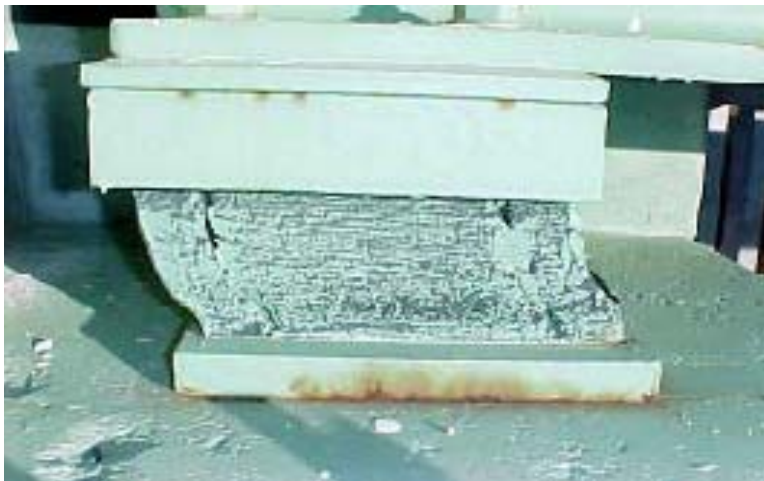
Figure 51 No Damage. Movement of the elastomeric bearing under thermal loads. (13)
