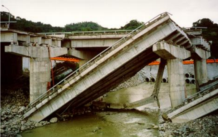
Figure 29 Total Failure. Collapse of simply supported precast, prestressed concrete girders. (4)
