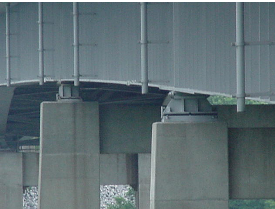
Figure 11 Continuous Welded Plate Girder Bridge (25)
