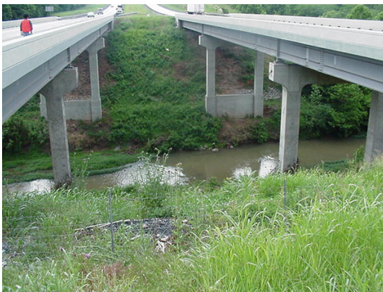
Figure 15 Welded Plate Girder Bridge (25)
