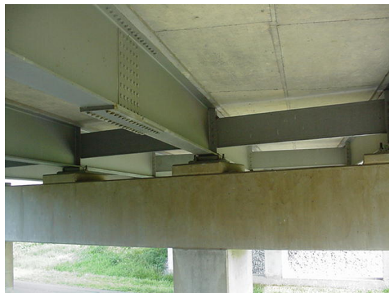
Figure 16 Welded Plate Girder Bridge (25)
