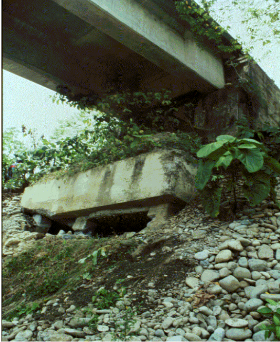
Figure 48 Severe Damage. Foundation movement. Longitudinal displacement and rotation of the abutment footing. Notice the flexure and shear failure of the exposed piles. (10)
