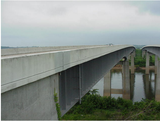
Figure 13 Welded Plate Girder Bridge (25)
