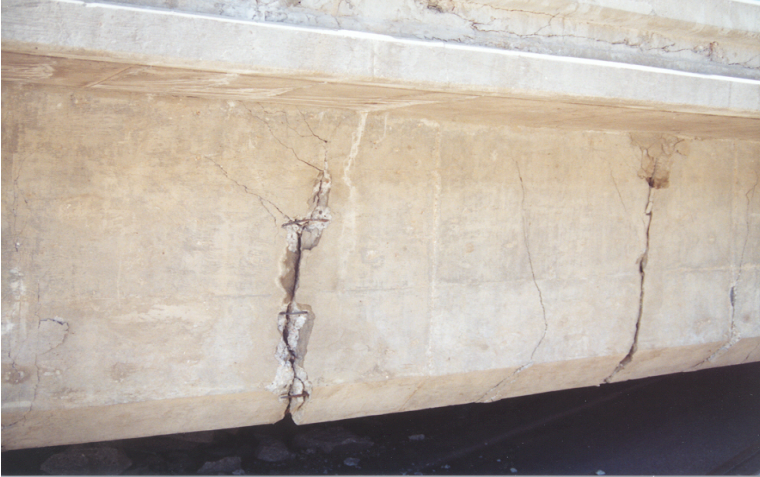
Figure 27 Moderate Damage. Flexural cracks in a concrete box girder bridge. (5)
