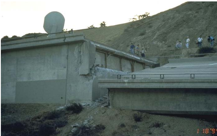
Figure 49 Total Failure. The shear key failed and the span unseated at the abutment. (1)
