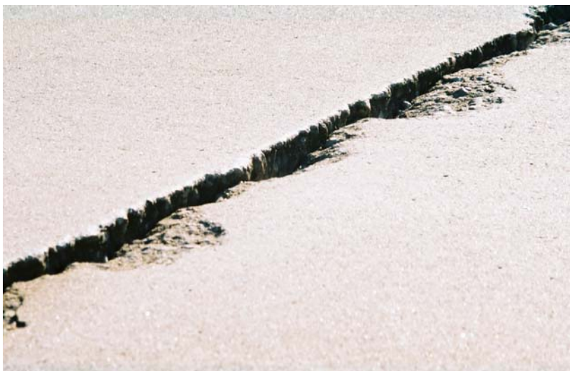
Figure 18c. Spall (Severe)
