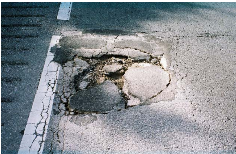
Figure 10c. Pothole (Severe)
