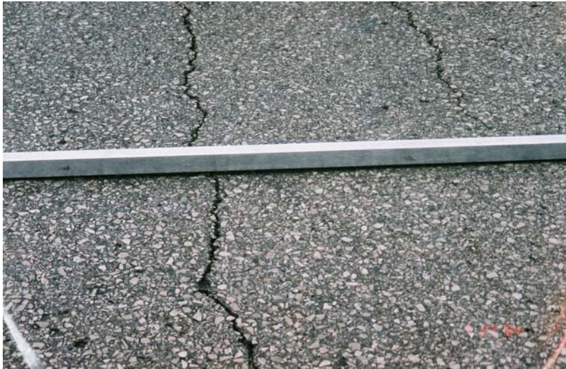
Figure 3a. Rutting (Slight)
