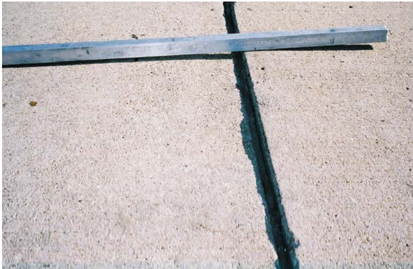
Figure 16a. Transverse Faulting (Slight)
