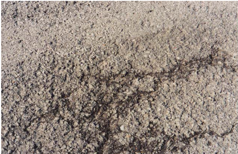
Figure 8c. Raveling (Severe)
