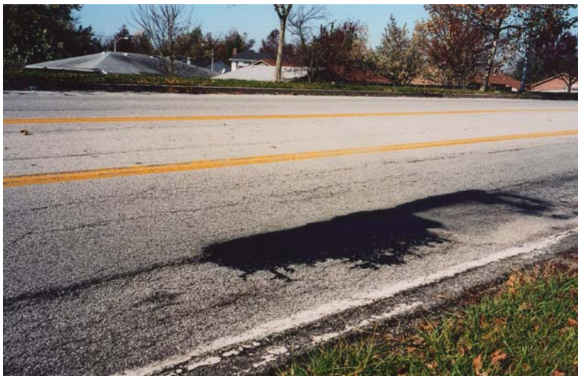
Figure 7c. Bleeding (Severe)
