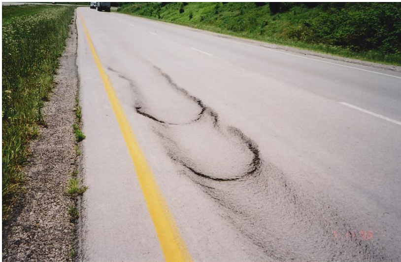
Figure 7c. Shoving (Severe)
