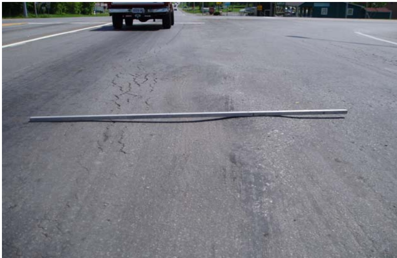
Figure 3c. Rutting (Moderate)
