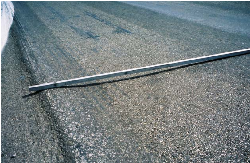
Figure 3b. Rutting (Moderate)
