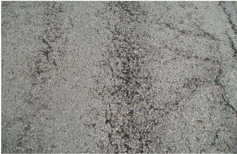
Figure 8b. Raveling (Moderate)
