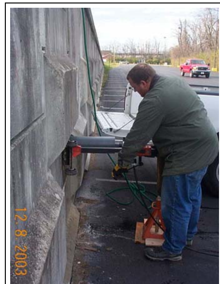
Figure 5. Coring an Access Hole.
