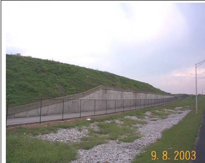
Figure 13. MSE Wall at Bluegrass Airport; Lexington, Kentucky
