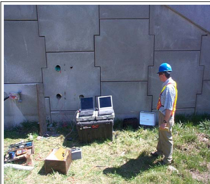
Figure 6. Corrosion Monitoring of a MSE Wall.
