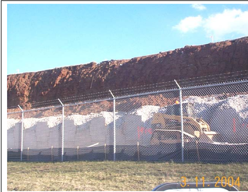
Figure 14. Demolition of an MSE Wall at Bluegrass Airport; Lexington, Kentucky.
