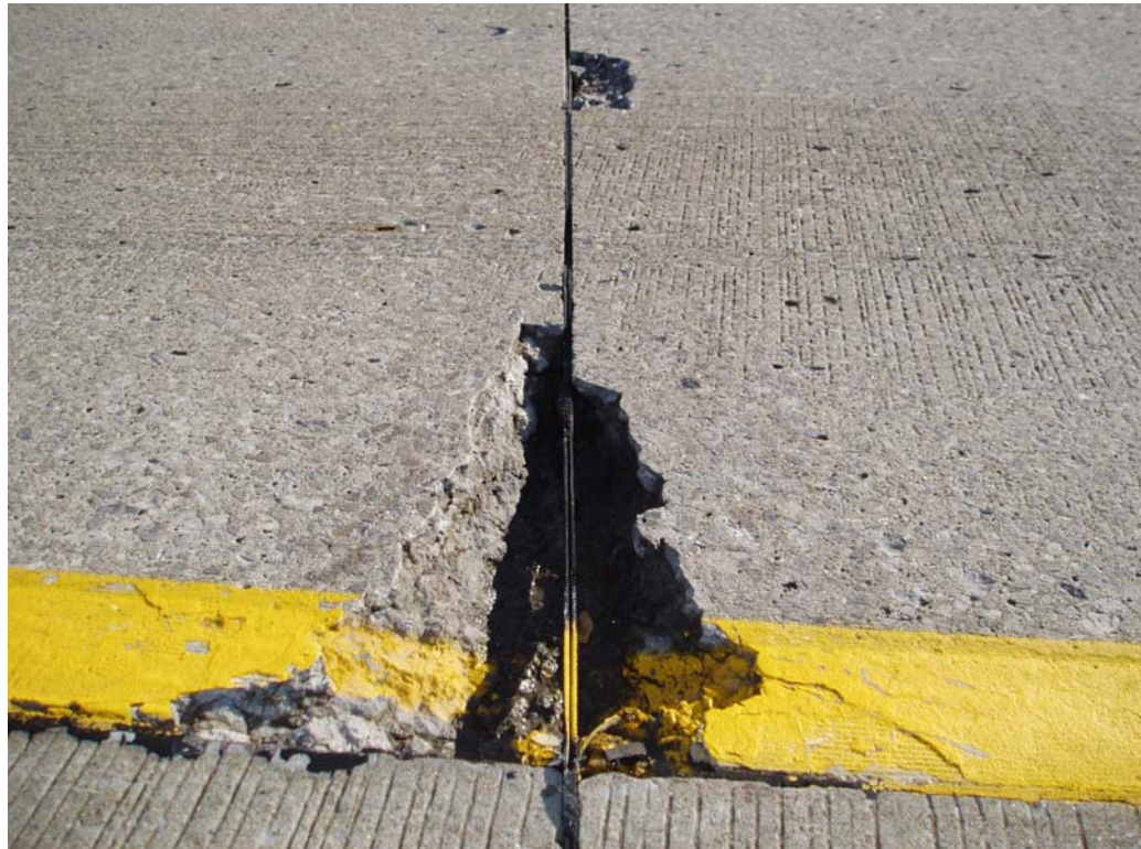
Figure 13: Spalled Joint
