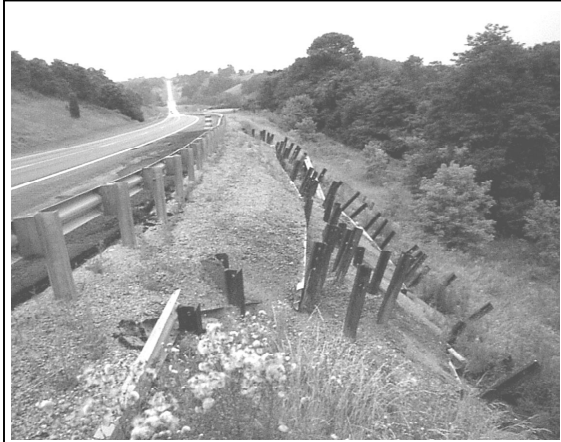
Figure 106. Past maintenance activities at a landslide site on US 68 in Mason County included driven rails that failed to arrest movements.
