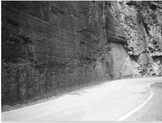
Figure 101. Rock slope on KY 80, MP 5.82 to 6.03, in Pike County.
