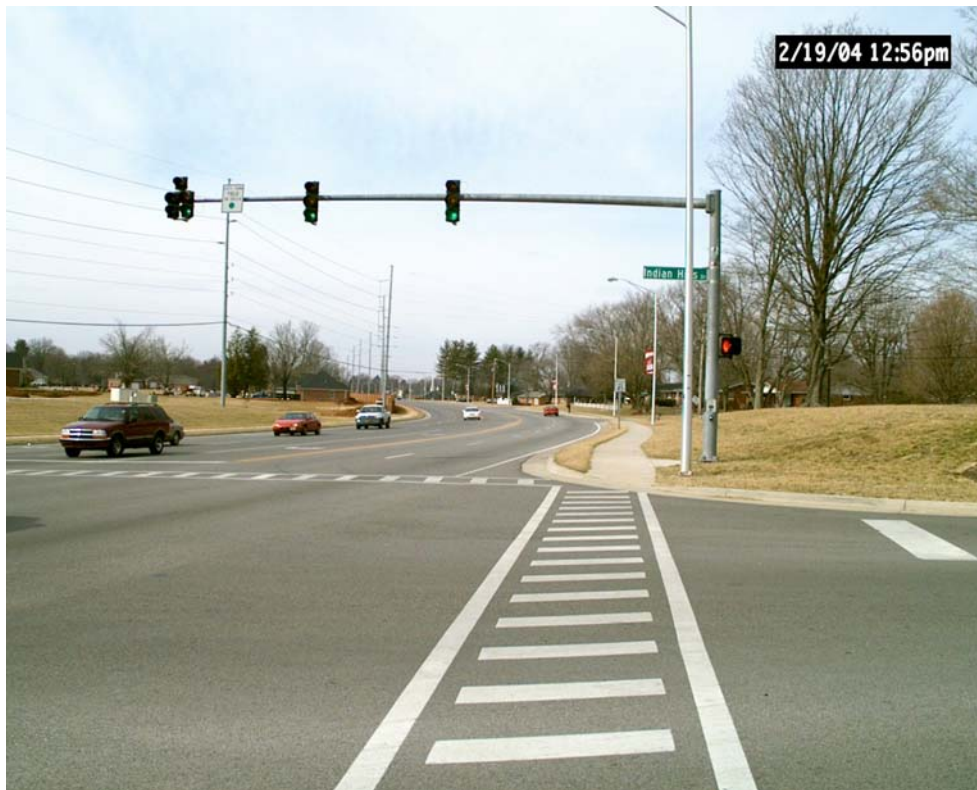
Figure 4. Sign pole and mast arm light signals were installed at four intersections along Cemetery Road/KY 234.
