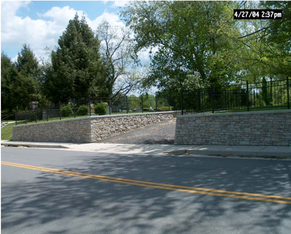
Figure 5. Rock facings were used on retaining walls in Perryville along U.S. 150. This is the front entrance into the Perryville Cemetery near the downtown area.
