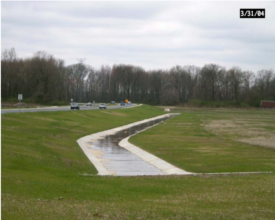
Figure 3. The permanent drainage system along Jefferson Boulevard is shown with wetland areas in the background.
