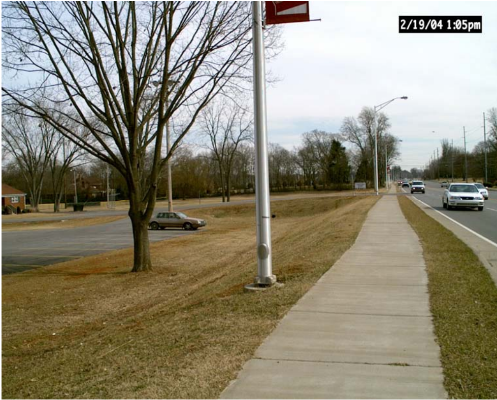
Figure 5. A small portion of Spero Keriakes Park was taken for ROW during the Cemetery Road/KY 234 project. A berm was used to transition between the park and sidewalk.
