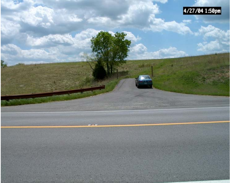
Figure 1. This is a typical paved farm entrance constructed along U.S. 150 by KYTC. Note the wide radius employed to facilitate use of the entrance by vehicles towing trailers.
