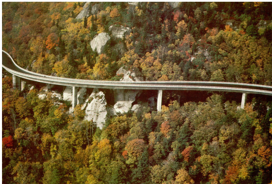
Figure B. Lynn Cove Viaduct Erected above Ground Level (Minimization).
