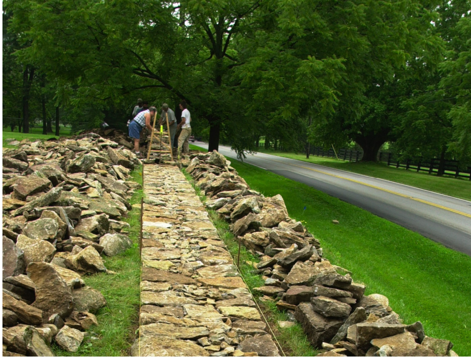
Figure C. Conservation Group Rebuilding a Dry Stone Fence (Mitigation).
