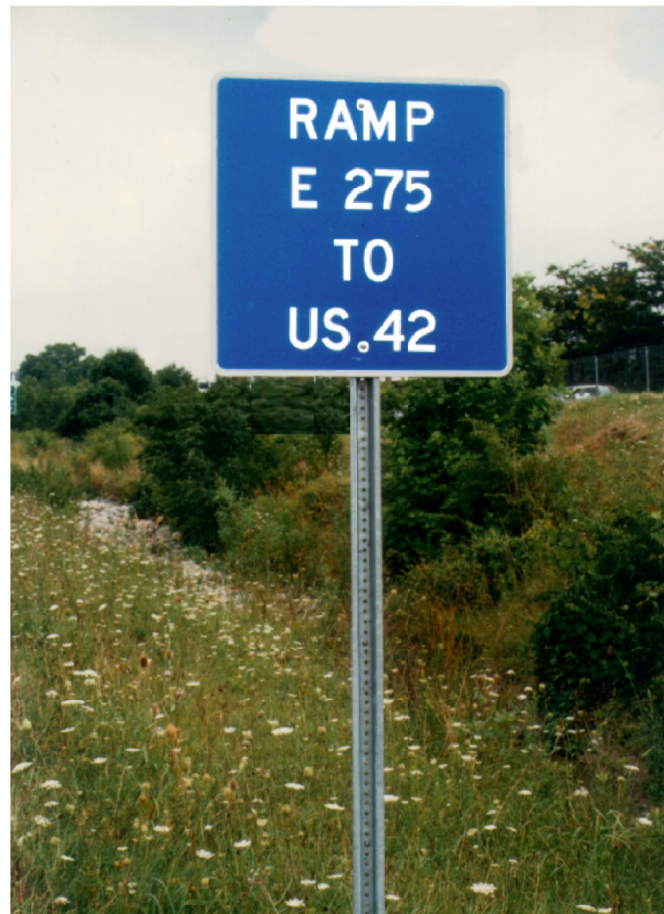
Figure 5. Photograph of Ramp Marker Used in the ARTIMIS Project.
