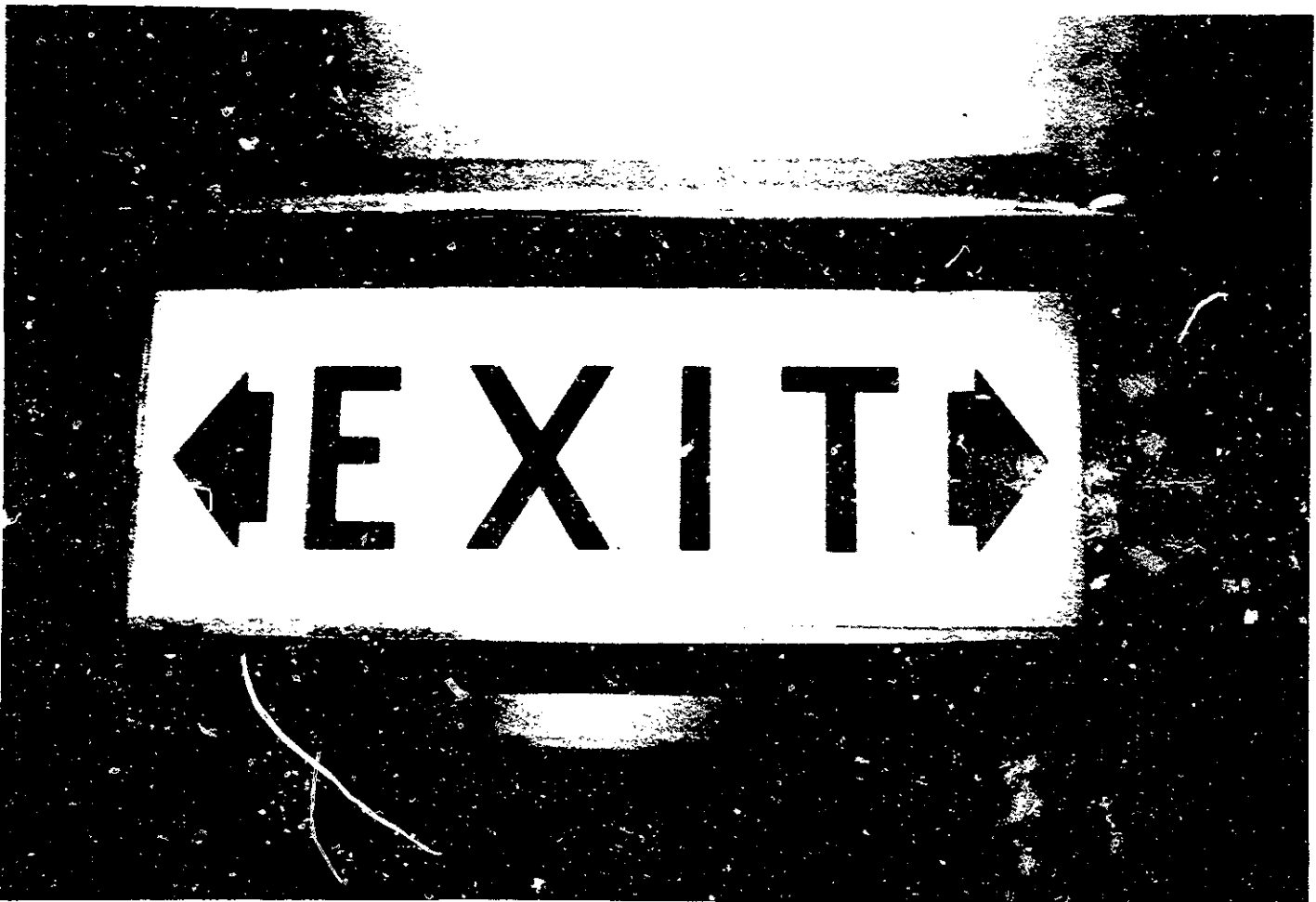
Figure 5. Cross-aisle exit locator sign mounted above the intersection of main and cross aisle at ceiling height.
