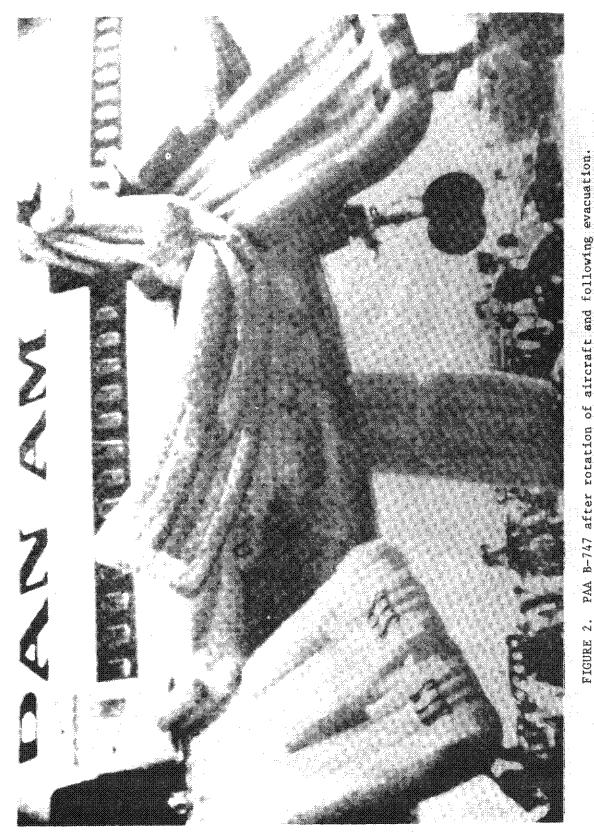
PAA B-747 after rotation of aircraft and following evacuation. Slides at the right and left front doors, number 2 exit slide, and slide at lounge area exit are shown.
