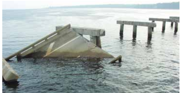
Top right: Within 14 days, two-way traffic was restored on the westbound I-10 bridge across Escambia Bay; misaligned decks are visible on the eastbound span.
