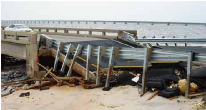
Top right: Within 14 days, two-way traffic was restored on the westbound I-10 bridge across Escambia Bay; misaligned decks are visible on the eastbound span.
