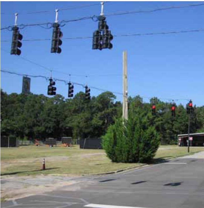
TERL's first test intersection is equipped with span-wire hanging traffic signals, traffic controllers, in-ground inductive-loop vehicle sensors, and closed circuit TV vehicle detection cameras.
