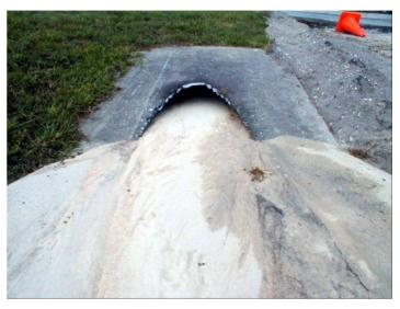
Uncontrolled erosion can result in blocked drainage systems.
