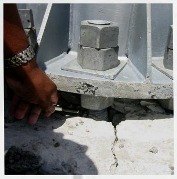
Cracks in the cement base can result in loosening of the pole supports, as shown here.
