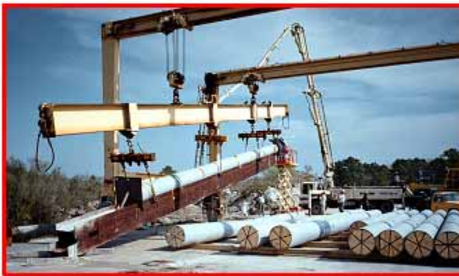
(b) Rear end showing wooden plugs
