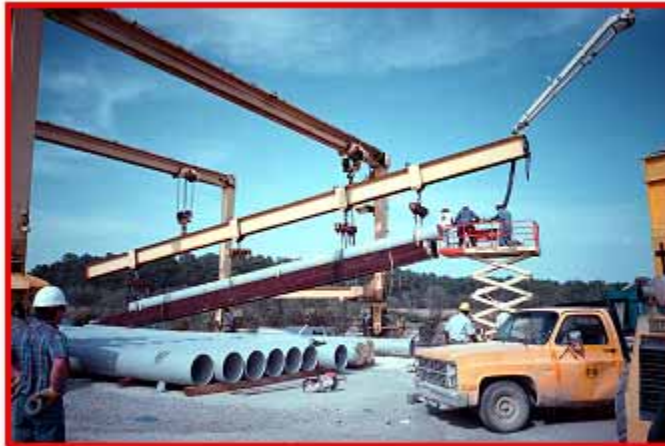
(a) Pumping concrete into the upper end
