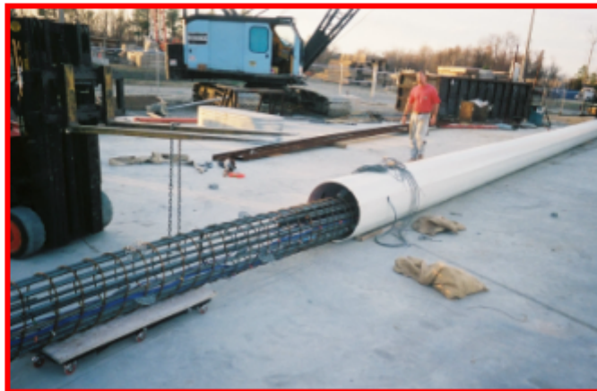
(c) Insertion of instrumented rebar cage into FRP tube
