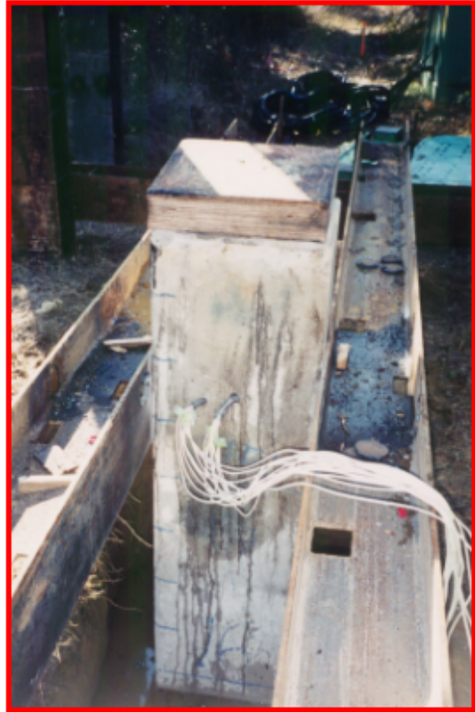
b) End of driving of prestressed pile showing driving cushion compressed
