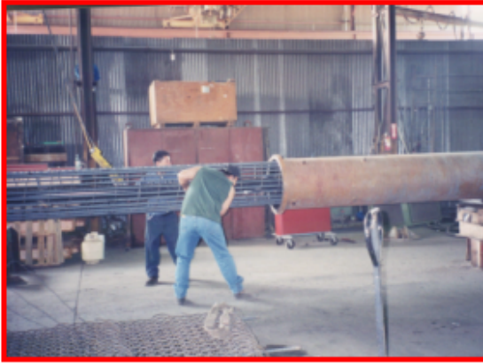
a) Instrumented rebar cage is inserted into steel mold
