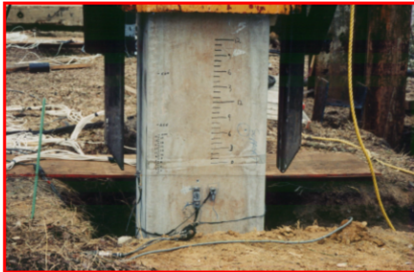
c) Restrike of prestressed pile
