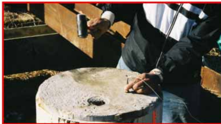
c) PIT on FRP pile after installation
