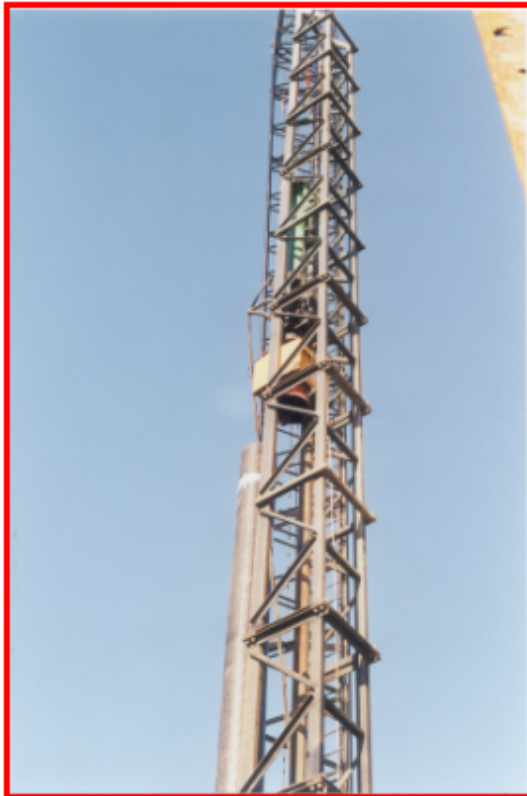
a) Driving of plastic pile
