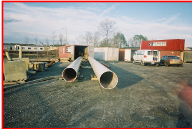
(a) FRP tubes received at the precast plant
