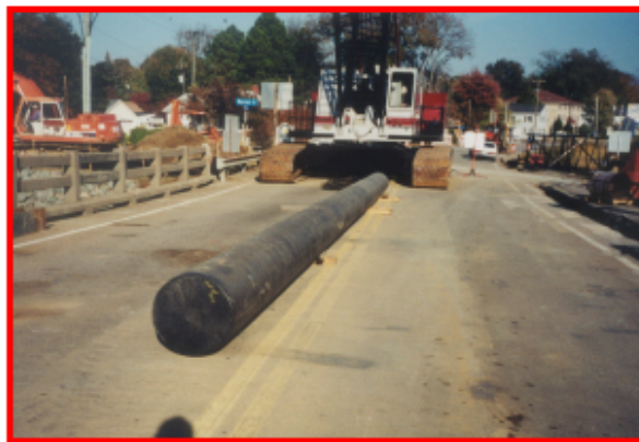
e) Finished plastic test pile
