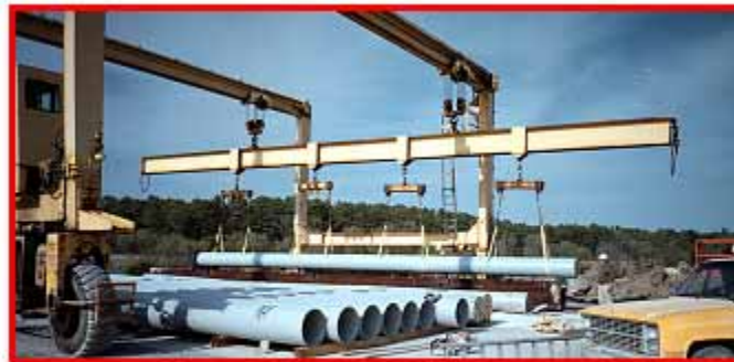
(c) Handling of the pile using 8-point supports
