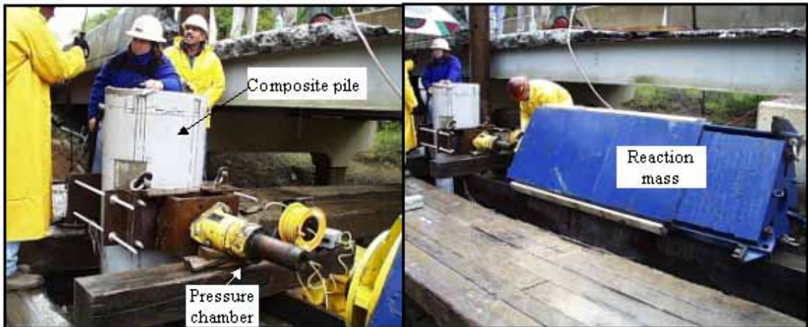
Figure 95. Photos. Lateral Statnamic setup at the Route 40 project.
