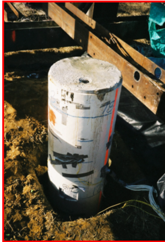
b) End of driving of FRP pile
