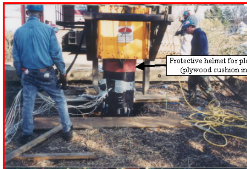
c) Restrike of plastic pile
