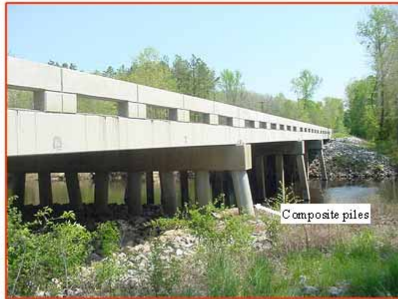
Figure 104. Photo. The new Route 40 Bridge over the Nottoway River in Virginia.
