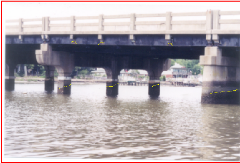
Figure 108. Photo. Signs of deterioration of the original Route 351 Bridge.
