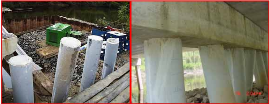
a) Photograph of composite piles installed at Pier No. 2 of the Route 40 Bridge
