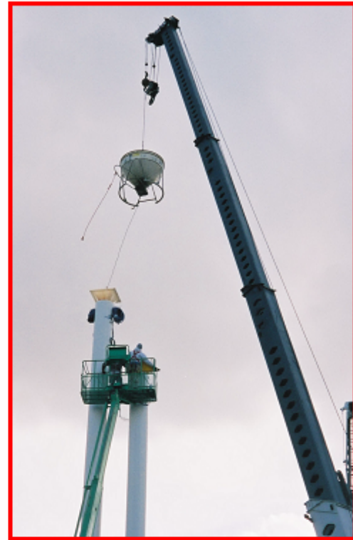
(b) Bucket with concrete is positioned over the pile with crane
