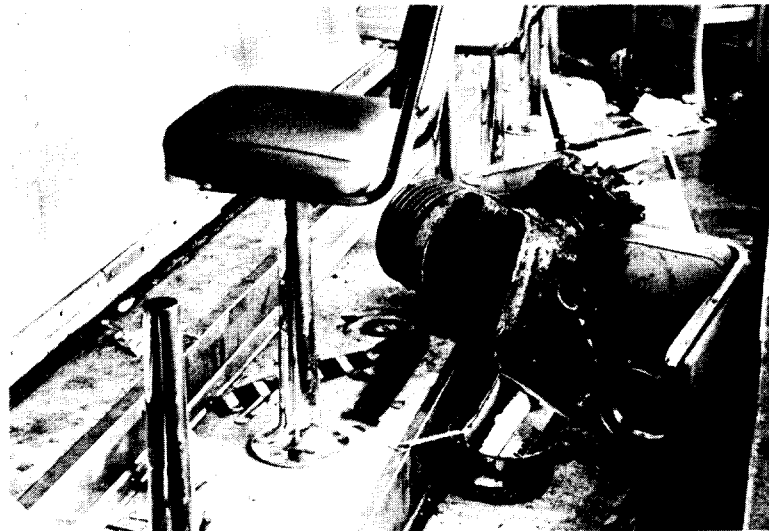
FIGURE 14. A heavy compressor penetrated the roof of the Diner just above the counter service area and broke off one of the stools at the counter.
