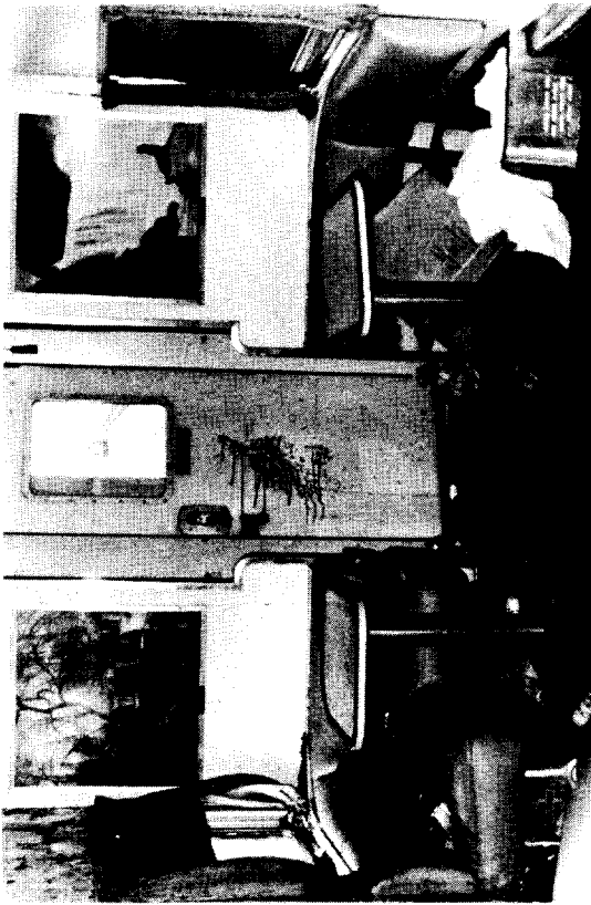
a. Front end of diner as it appeared with car on its side. Passengers escaped by climbing up on the booth and out the end door.
