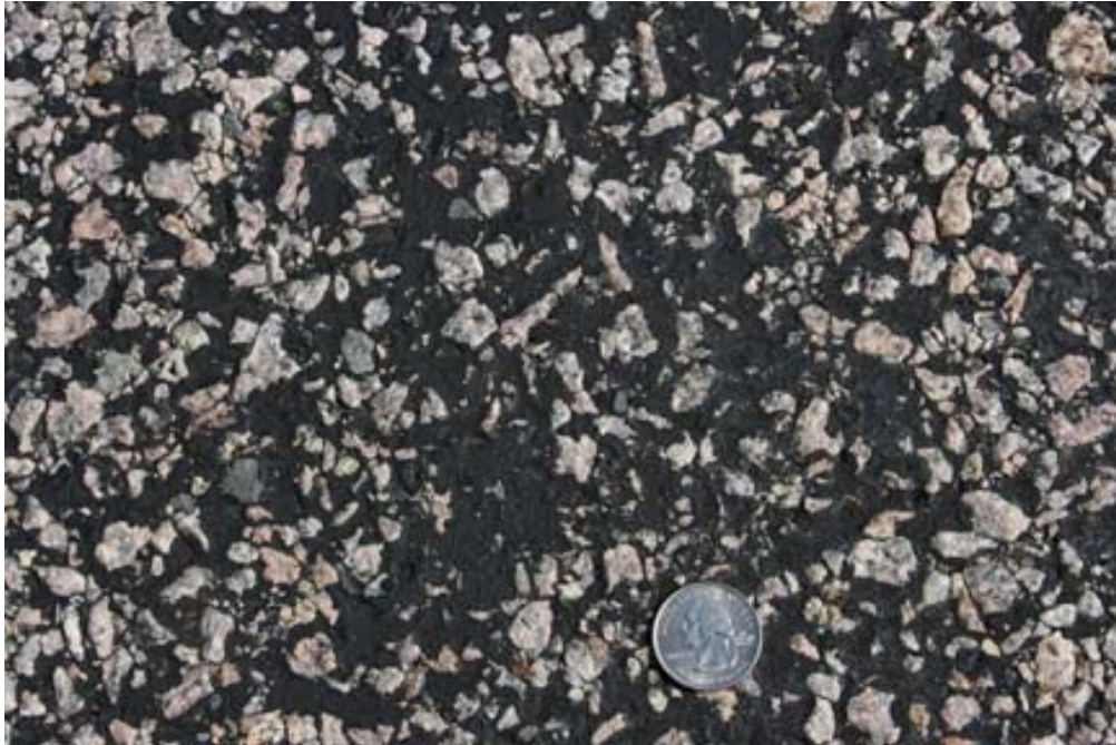
Figure 7-1 Flushed surface texture of single seal in Section 5 with granite 78M and CRS-2 emulsion
