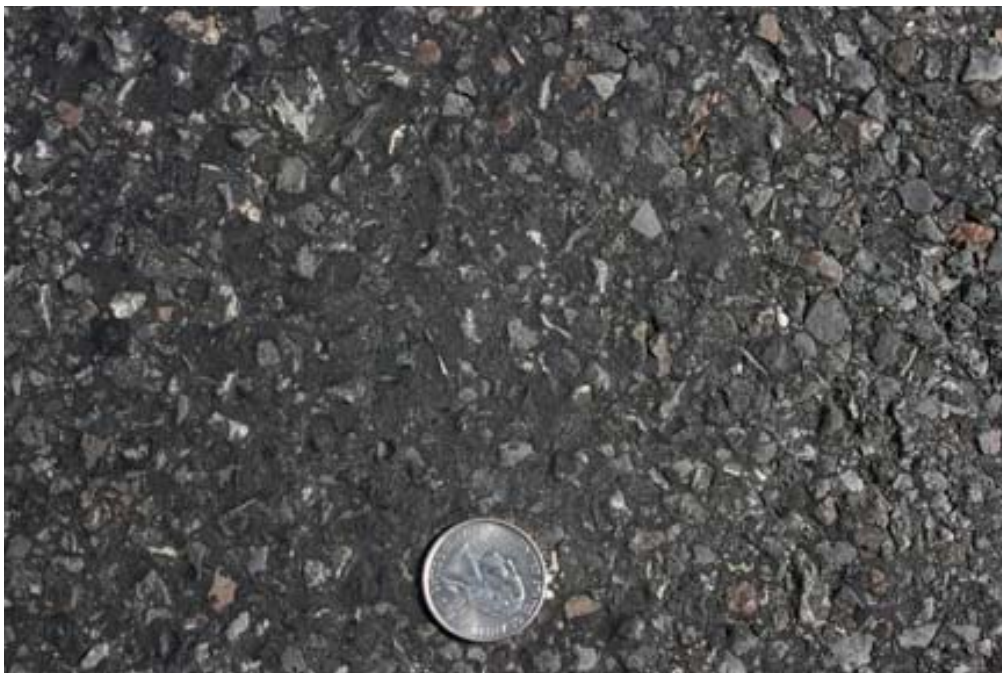
Figure 7-2 Flushed surface texture of double seal (78M/Lightweight) in Section 3 with CRS-2 emulsion
