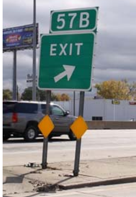
Figure 24. Reflective Object Markers on Sign Posts.
