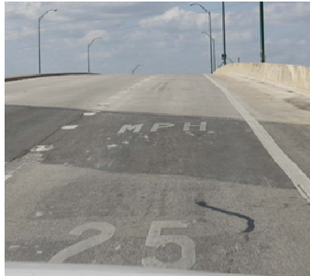
Ramp speed painted on the pavement
