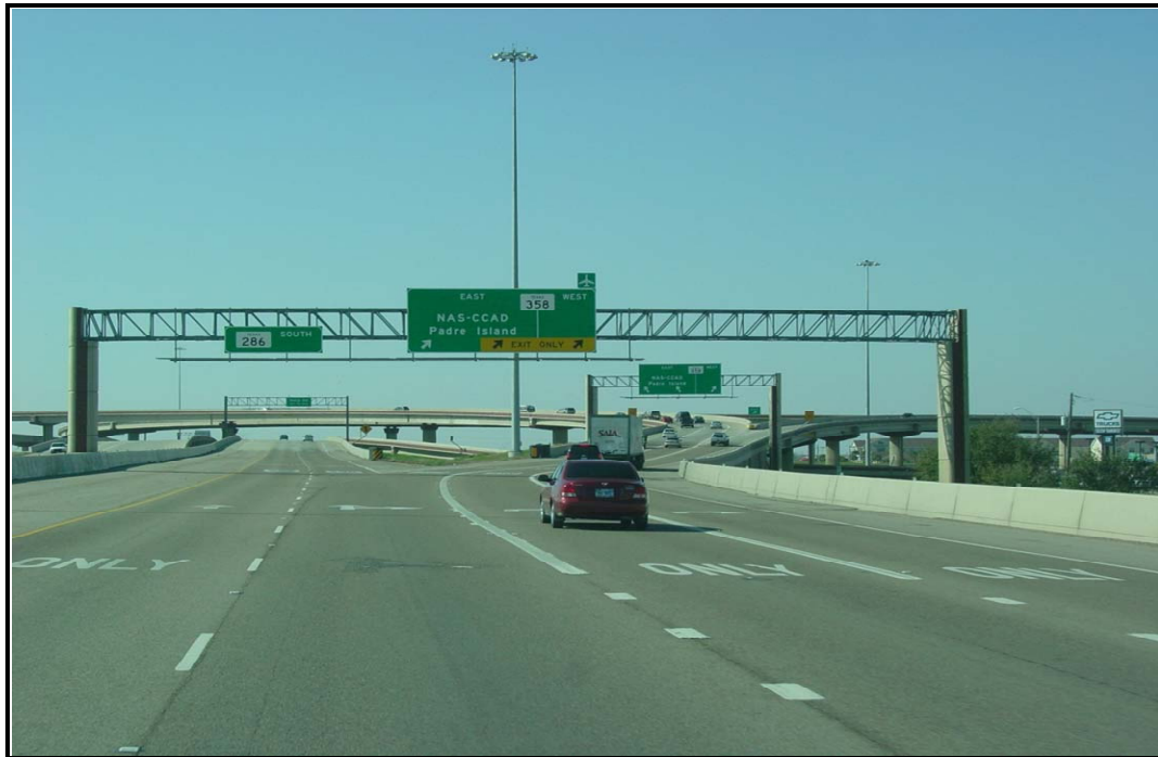
Figure 26. Southbound SH 286 Exit to SH 358 East, Corpus Christi, Texas.
