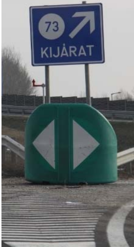
Figure 23. Impact Attenuator with Large Retro-Reflective Bi-Directional Arrows.
