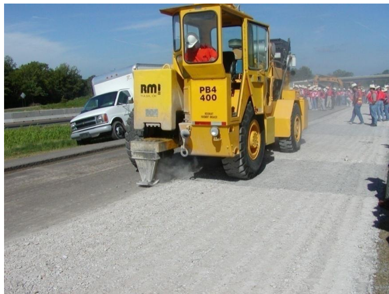
Figure 8 Resonant Pavement Breaker
