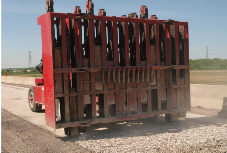
Figure 35 Rubblization Using Specialties MHB
