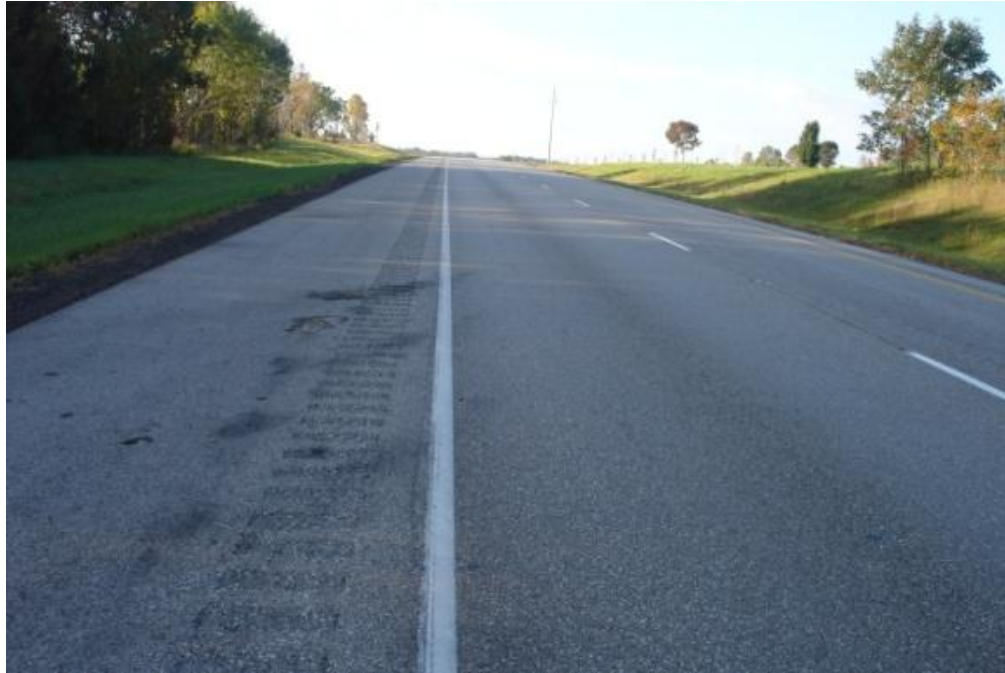
Figure 13 Typical View of MED 271 Section
