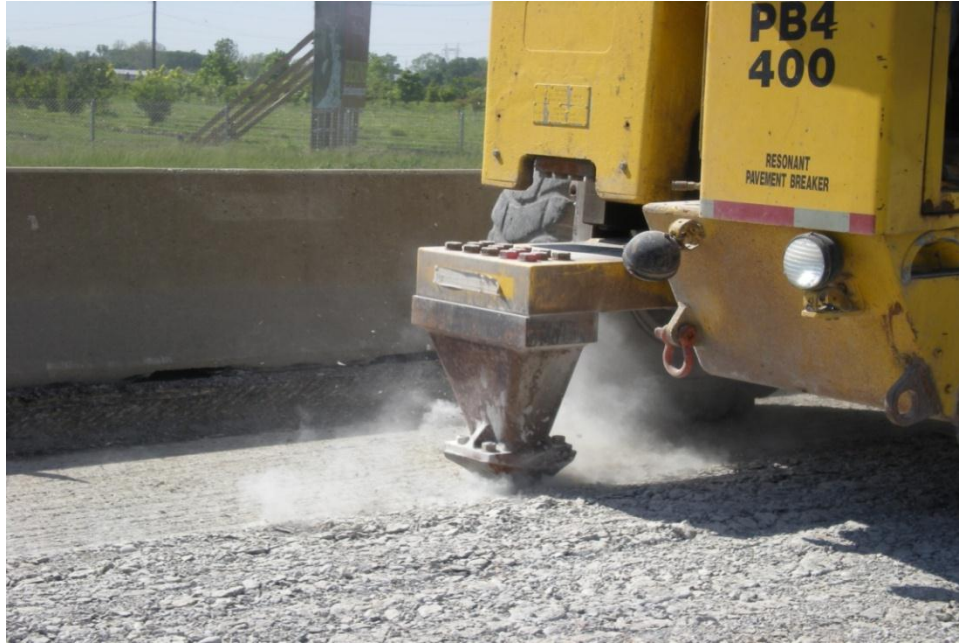
Figure 33 Rubblization Using RPB
