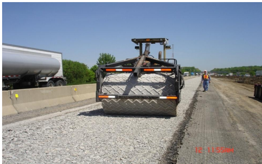
Figure 38 Rolling With a Vibratory Steel roller
