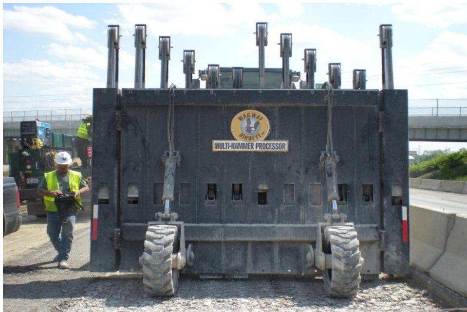
Figure 36 Rubblization Using Wagway MHB
