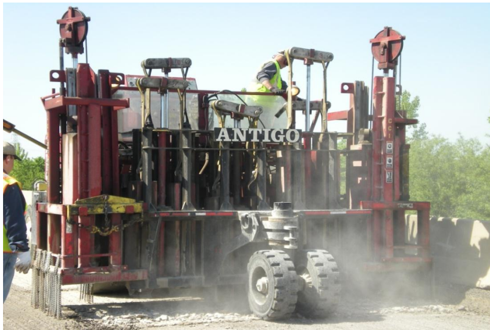
Figure 34 Rubblization Using MHB Badger Breaker
