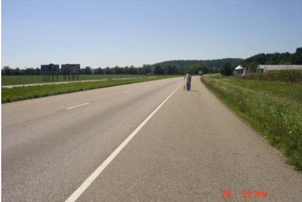
Figure 11 Typical View of COS 36 Section
