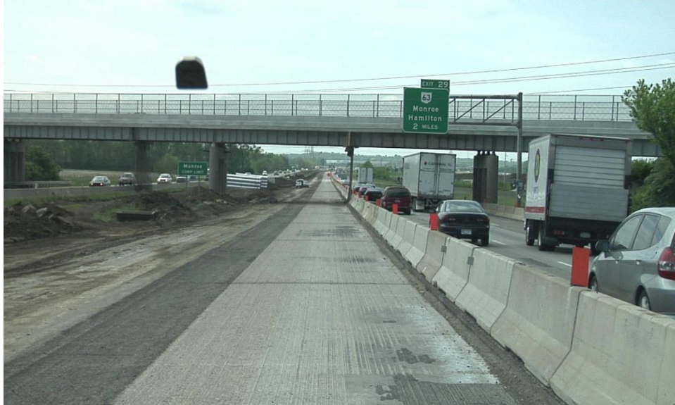
Figure 32 Asphalt Layer Milled and Prepared for Rubblization
