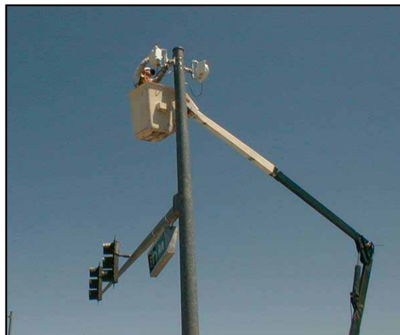
Figure 8-6: Installation of Wireless System - Photograph Courtesy GDI Systems, LLC
