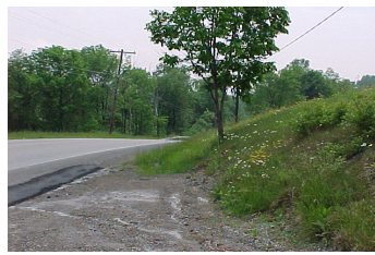
Before slope flattening
