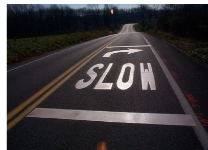
The advanced curve warning treatment warns drivers to reduce speeds.
