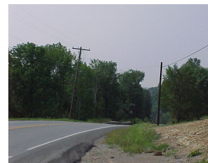
After slope flattening
