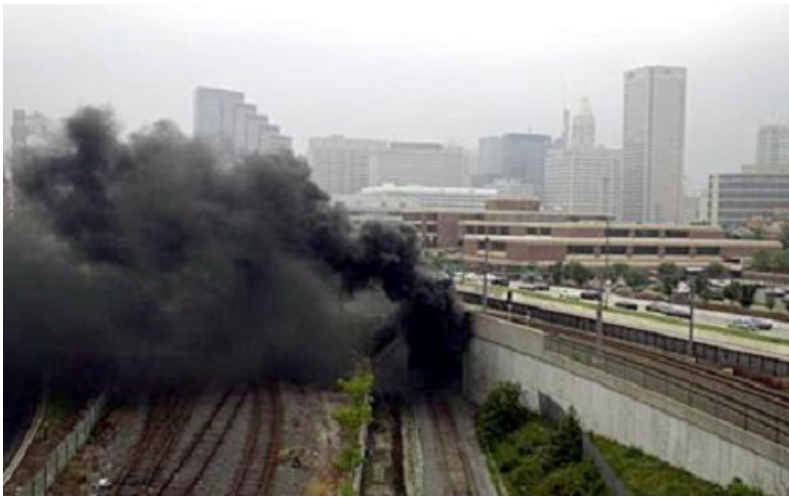
Figure 4. Smoke Billows from the Tunnel's South Portal, with the Baltimore City Skyline in the Background.
