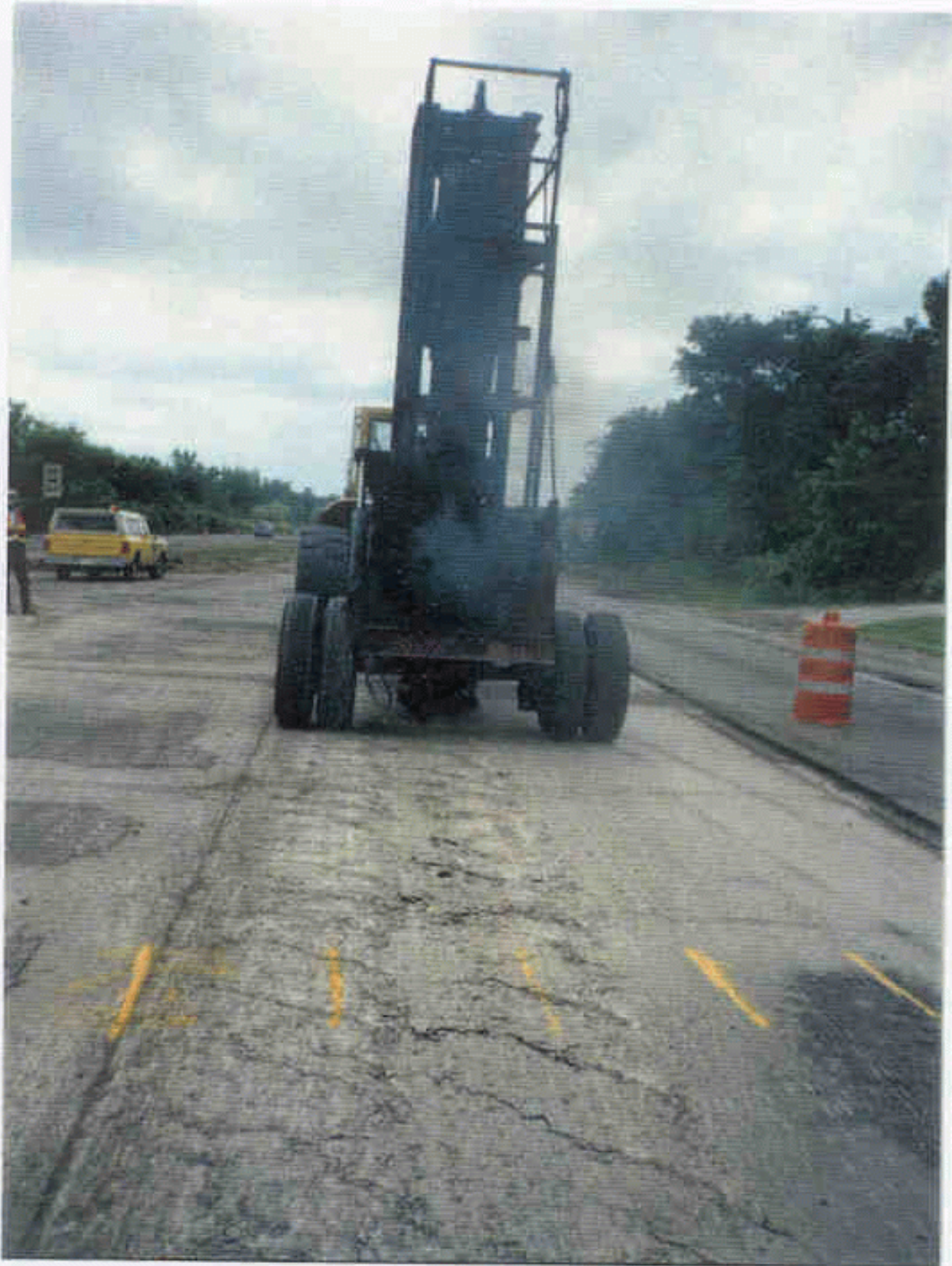
Figure 2. Pile Hammer in Operation on SR-4 Sections
