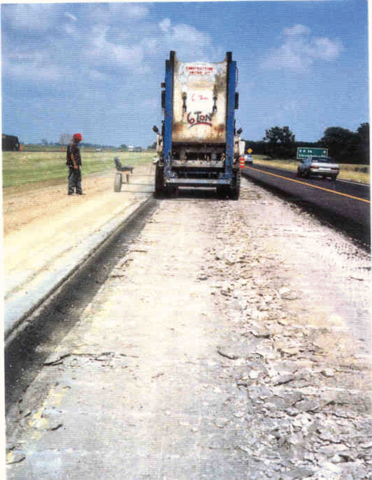
Figure 3. Breaking Pattern with Guillotine Hammer
