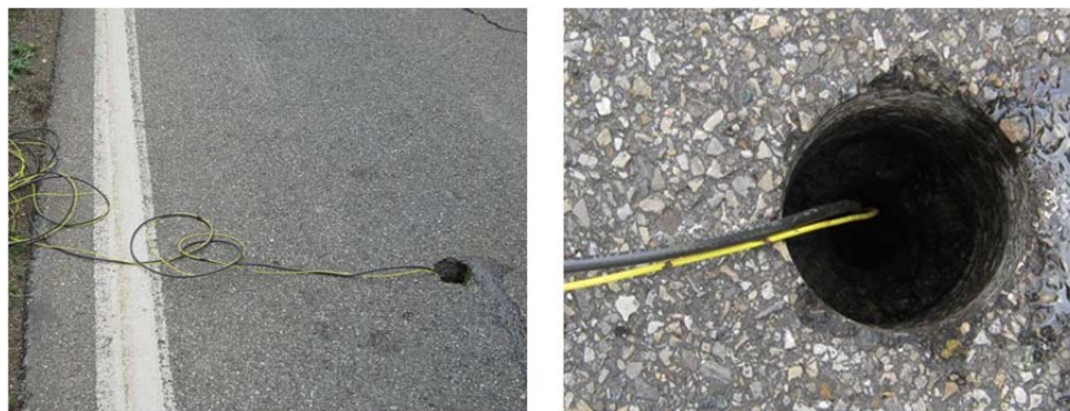
Figure 2.9. ATH 690-1 after the cone rods were pulled out and cables are being held by the disposable tip.
