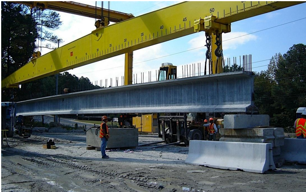
Figure 2-2: Load test set-up
