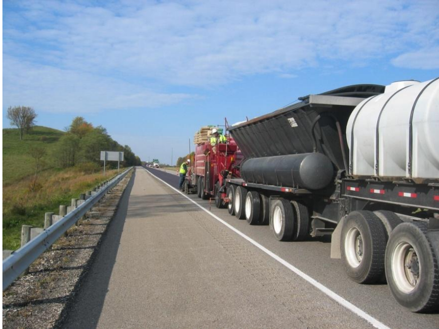
Figure 3. Micro Surfacing Treatment in Progress
