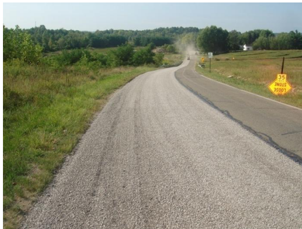
Figure 1. Chip Seal Treatment in Progress
