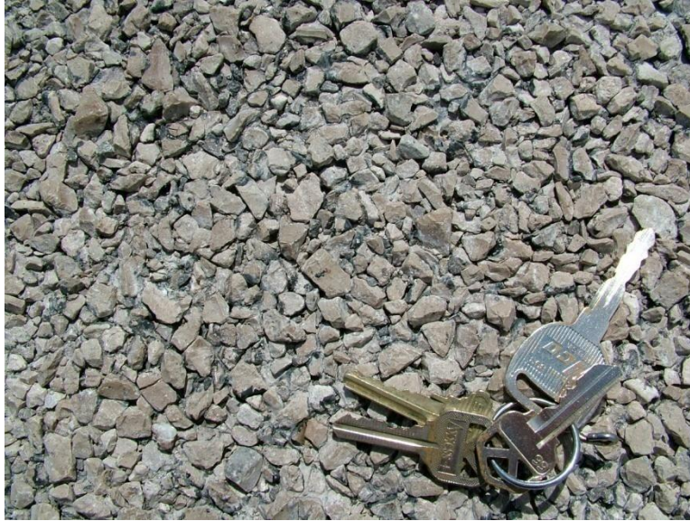
Figure 2. Close-up View of Finished Chip Seal Project
