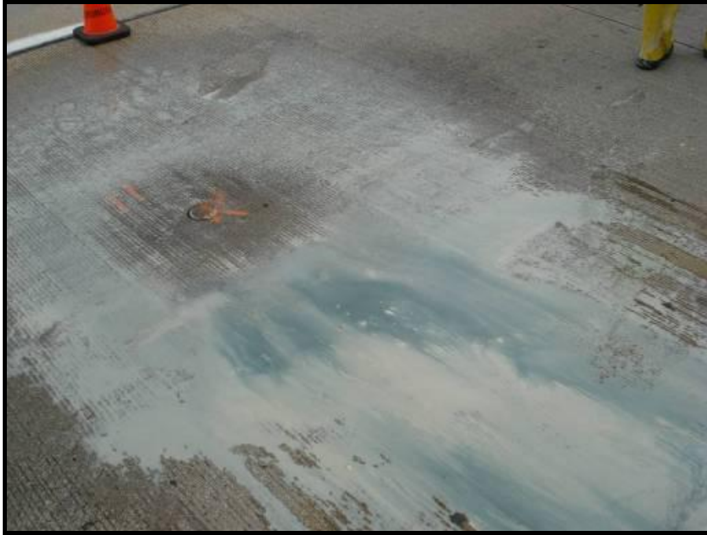
Figure F13. – Green Slurry from Slag Aggregate
