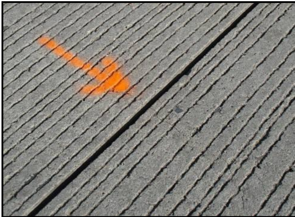
Figure F1. – Longitudinal Crack over Dowel Bar on ALL 30
