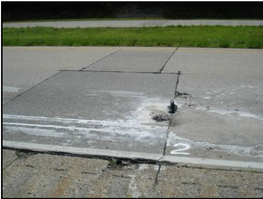
Figure F6. – Joint Replacements on ATH 33
