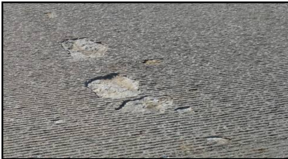
Figure F24. – Popouts from High Steel on GRE 35 19W
