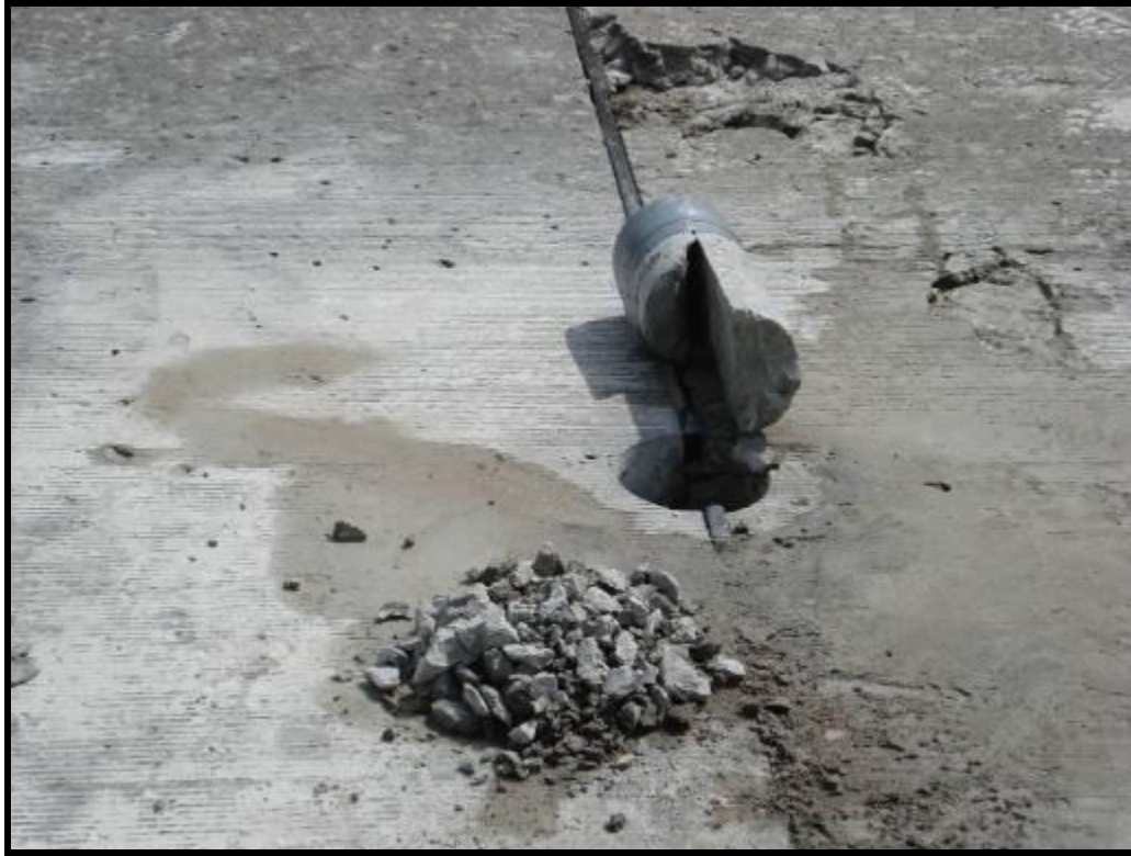
Figure F7. – Deteriorated Concrete in Joint Replacement
