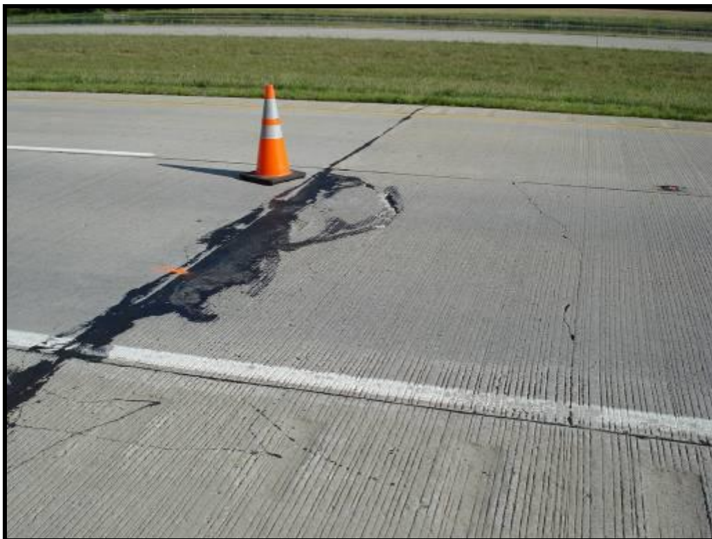
Figure F3. – Distressed Slab at Beginning of New Pour
