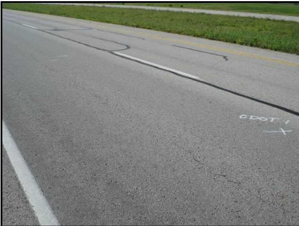
Figure E27. – Centerline Cracking
