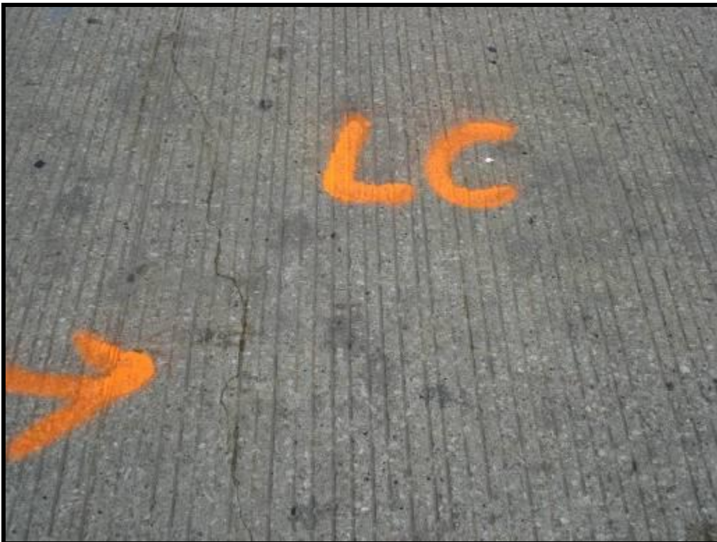
Figure F12. – Transverse Crack
