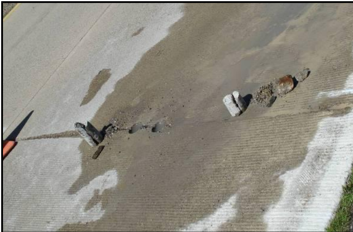
Figure F9. – Deteriorated Concrete at Bottom of Joint
