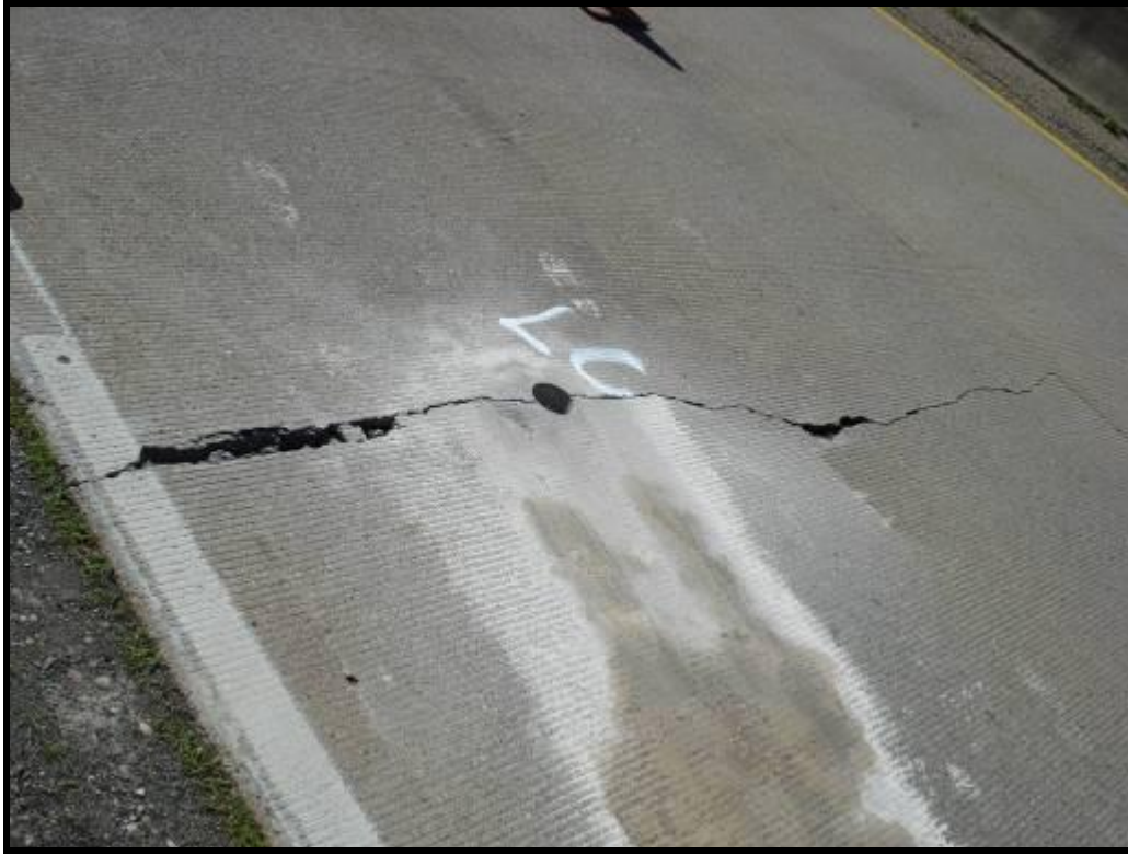
Figure F8. – Transverse Crack on ATH 682
