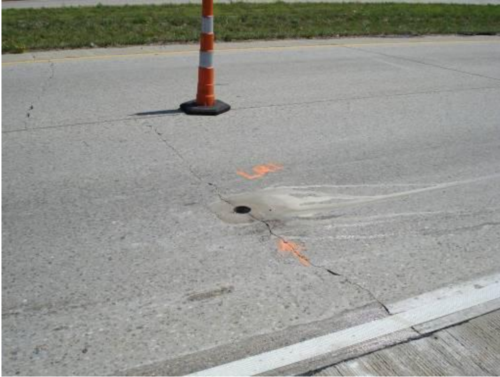
Figure F26. – Transverse Crack
