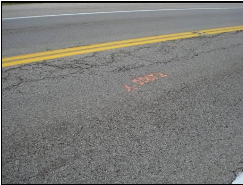
Figure E5. – Surface Cracking on CHP 68 2.5N
