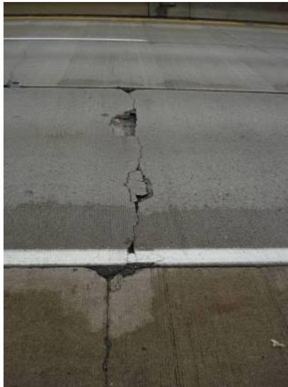
Figure F28. – Severe Transverse Crack
