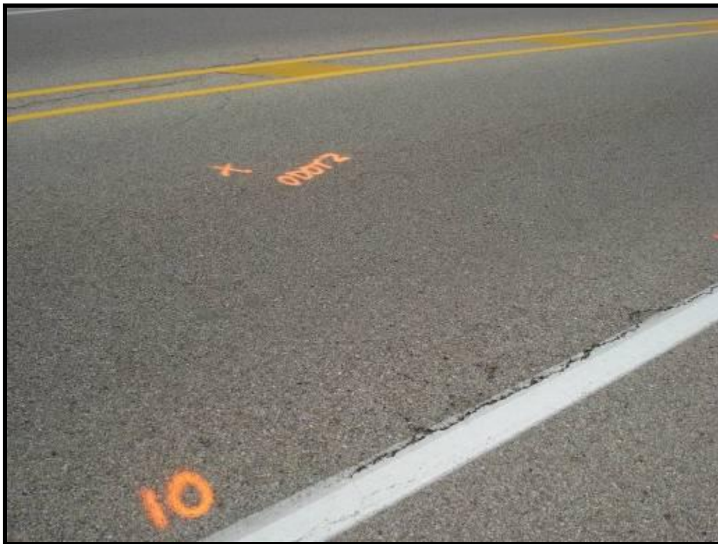
Figure E4. – Minor edge cracking on CHP 2 N
