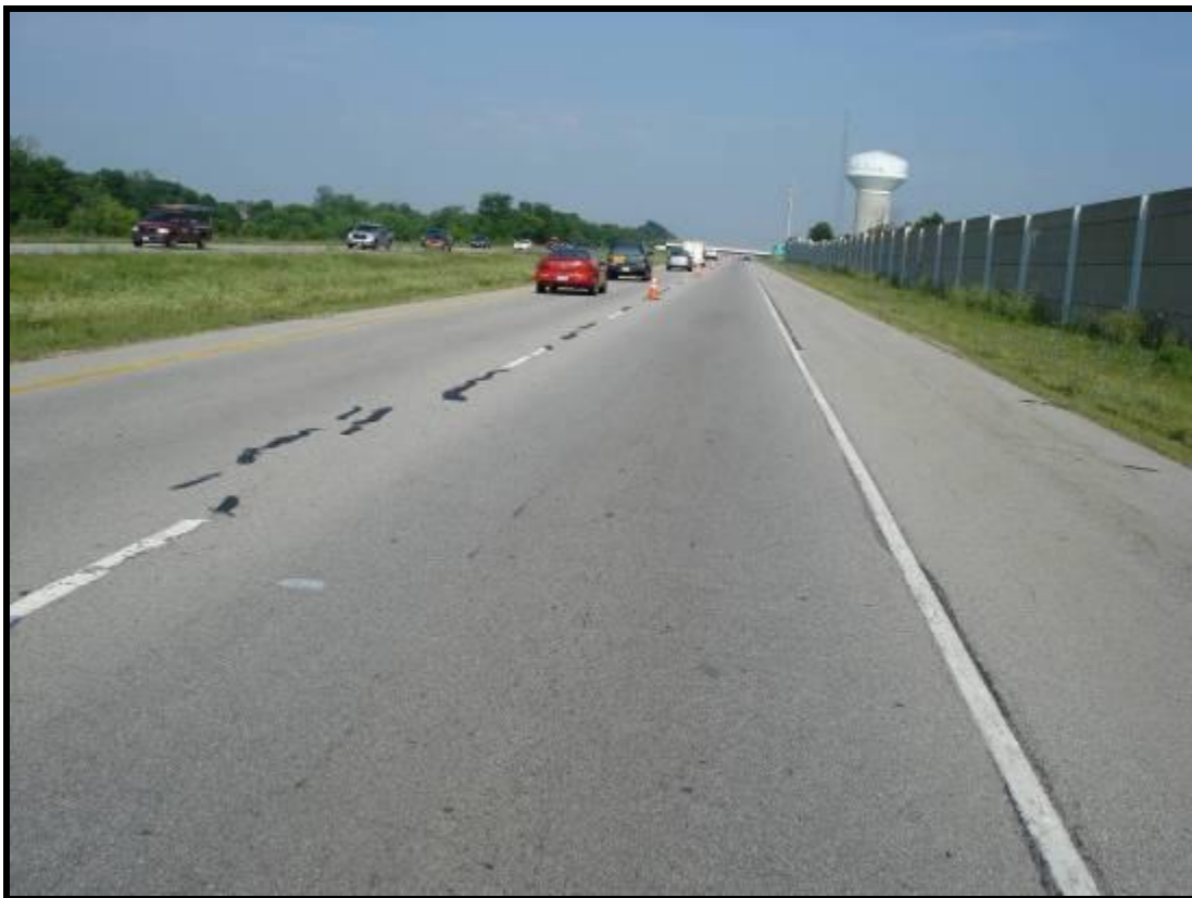
Figure E2. – Longitudinal Centerline Cracking on BUT 129 22 W
