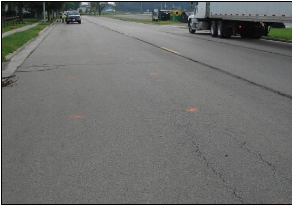
Figure E8. – Surface Cracking on CLA 41 3N
