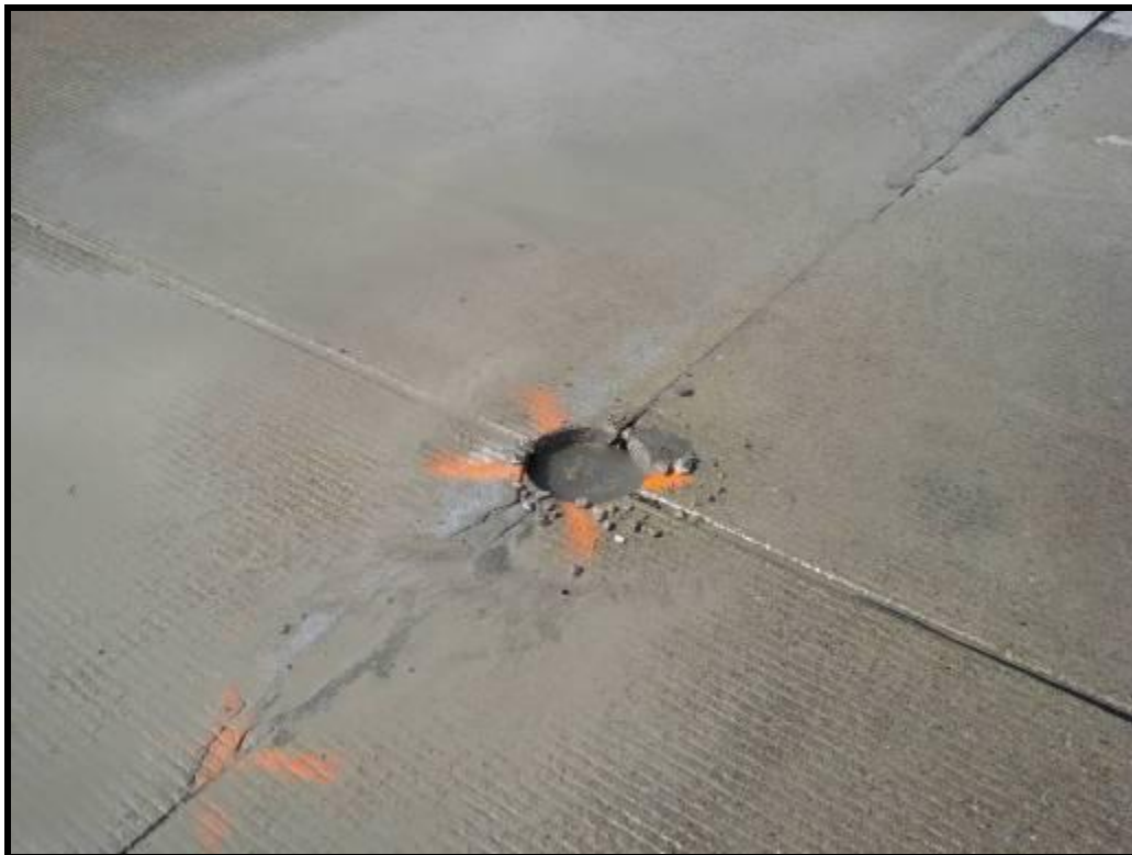
Figure F32. – Distress along Longitudinal Joint
