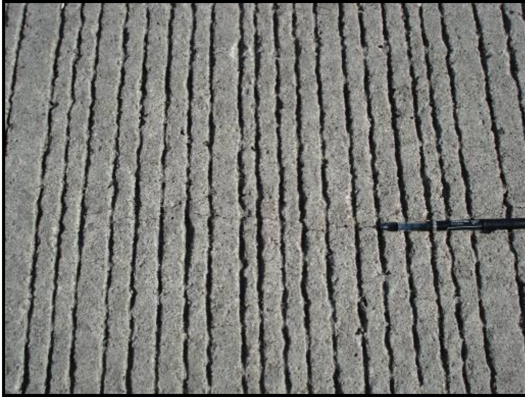
Figure F2. – Longitudinal Crack over Mesh Reinforcement
