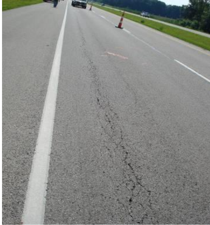
Figure E24. – Wheelpath Cracking
