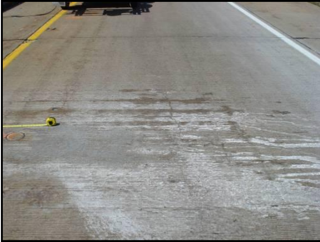
Figure F16. - Longitudinal Hairline Cracking in Center of Slab
