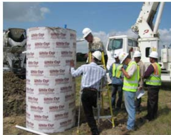
(b) 7 and 7.5 ft (2.1 and 2.3 m) Tall Sonotube Casing for Reaction Shaft
