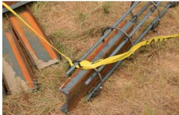
Figure 4.9. Channel Steel Tied to Steel Rebar Cage.
