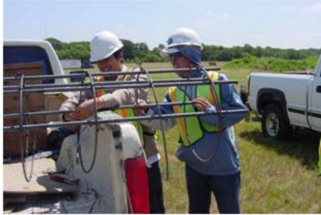
Figure 4.6. Construction of a Test Shaft Rebar Cage.
