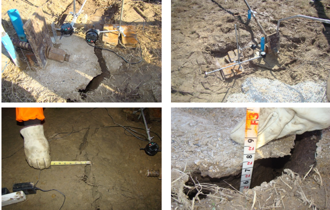
Figure 5.9. Test Shaft Displacement in Winter Condition.
