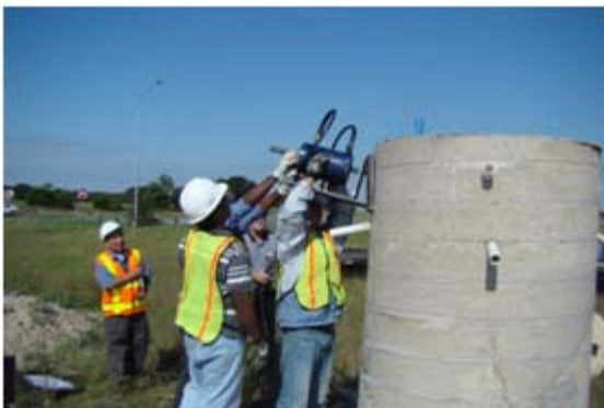
(a) Installing the Hydraulic Piston
