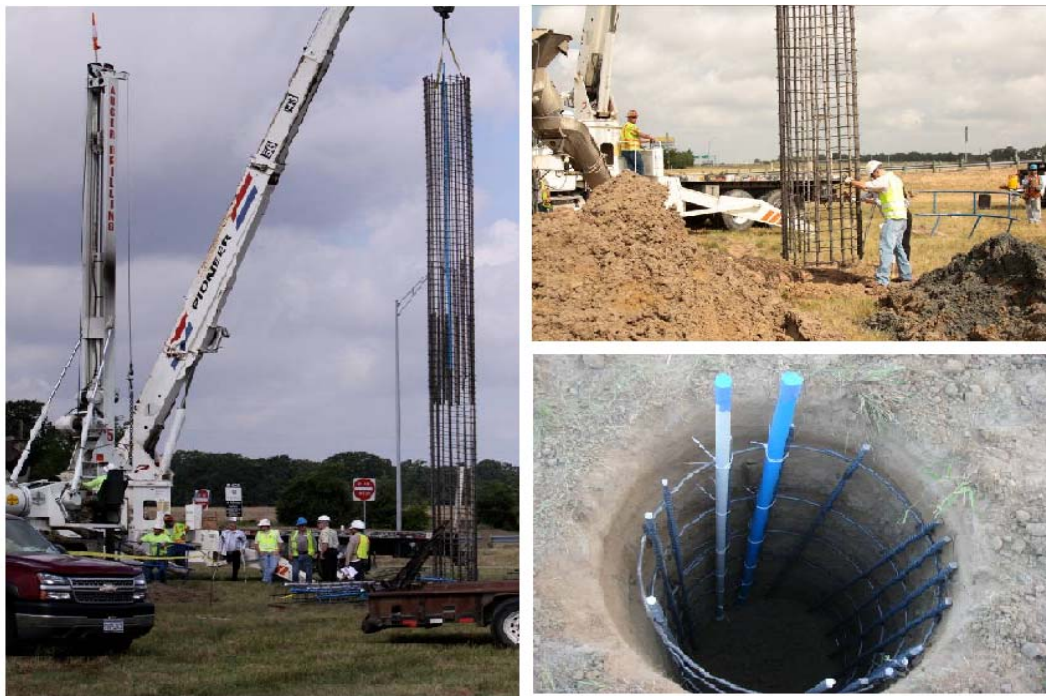
Figure 4.10. Setting the Steel Rebar Cages.
