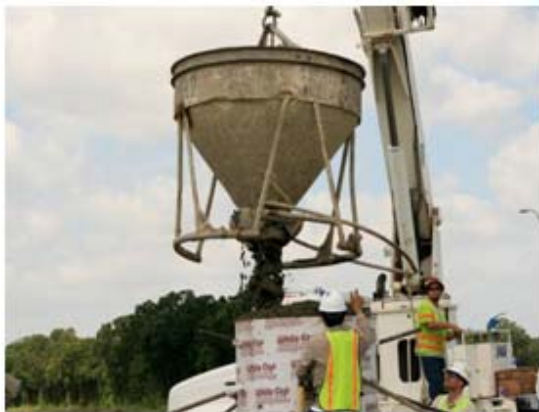
(a) Pouring Concrete in Sonotubes
