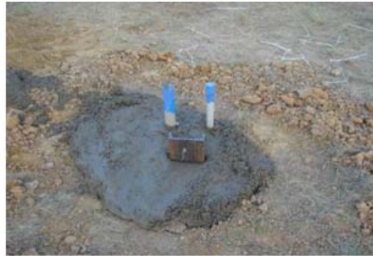
Figure 4.11. Pouring Concrete and Final Shaft.
