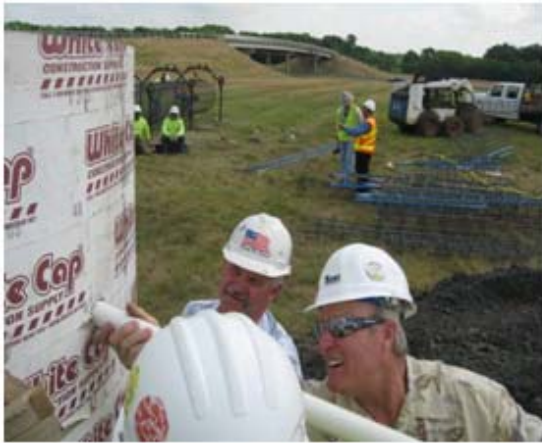
(a) Installing the PVC Pipe
