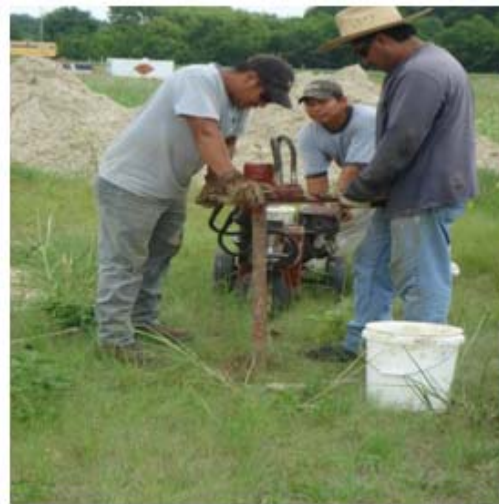
(b) Drilling Operation
