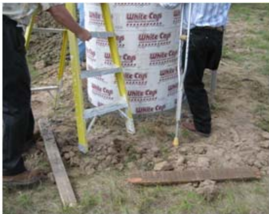
(a) Setting Sonotube casing for Reaction Shaft
