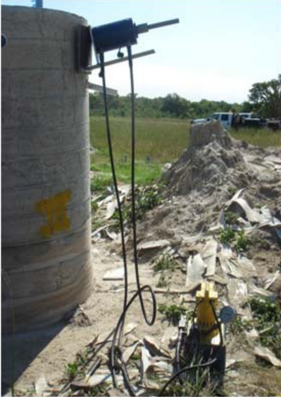
(a) Tensioning System Setup
