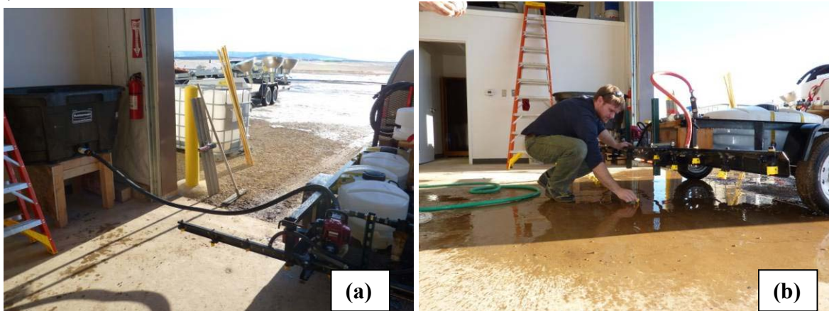
Figure 12 Raised tank filled with warm well water connected to the trailer to flush the system (a) and replacing clean nozzles for final flush with the next anti-icer (b).
