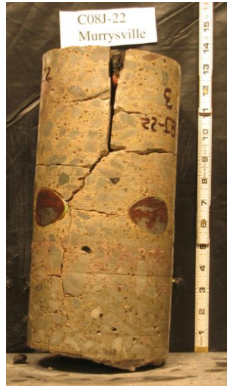
Figure 55: PCC Core Retrieved at the Transverse Joint of Slab 8 of US-22 Murrysville Segment 50 Eastbound.
