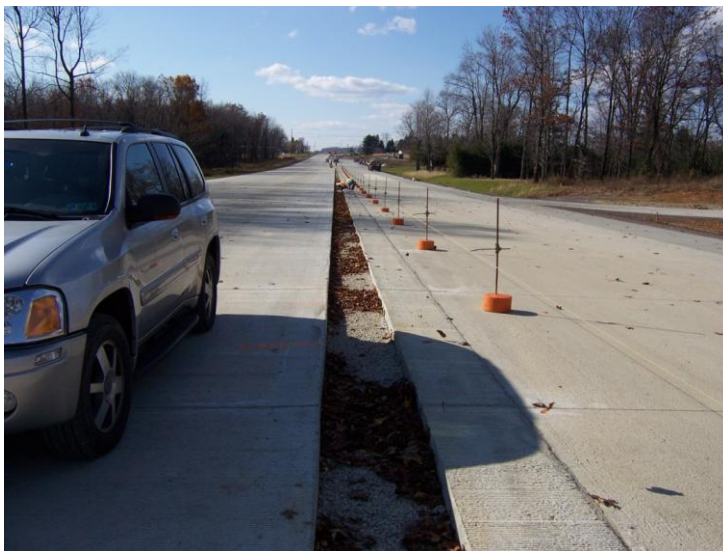
Figure 154: Overall View of US 22, Indiana County, Showing 2-ft Shoulder
