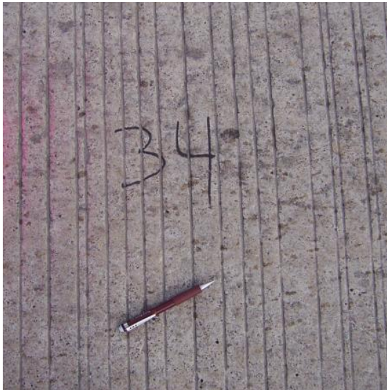
Figure 64: Overall View of Slab 34 US-22, Westmoreland County Segment 50 Eastbound
