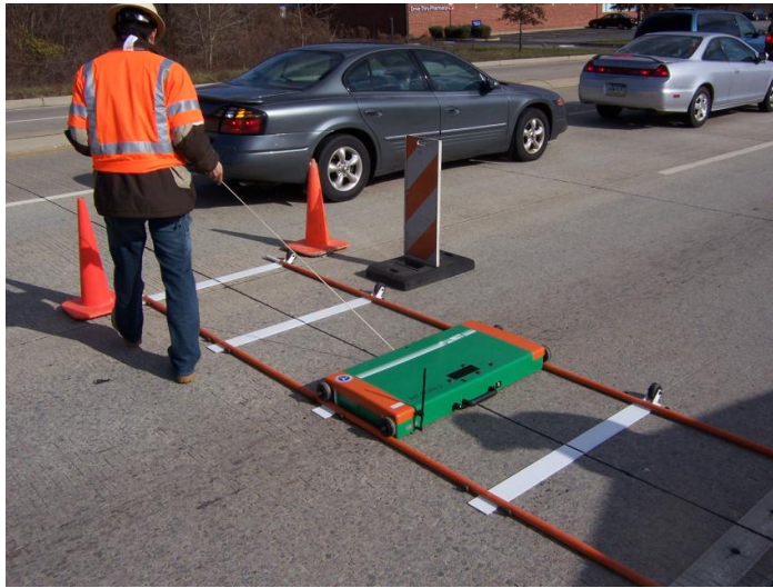
Figure 71: Dowel Scanning Using the MIT Scan-2 at US-22 Murrysville Segment 50 eastbound.
