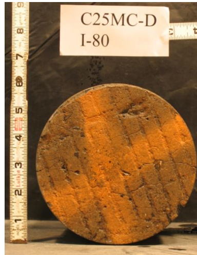
Figure 148: Top View of PCC Core Retrieved at a Microcracked Location of I 80 Segment 1914 Eastbound, Slab 25,(Distressed Section)
