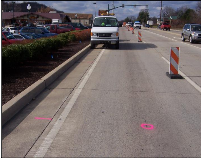
Figure 50: Overall Condition of US-22 Murrysville Segment 50 Eastbound.
