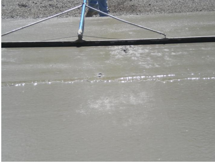
Figure 78: Slurry Produced by the Wet Burlap Drag behind the Paver
