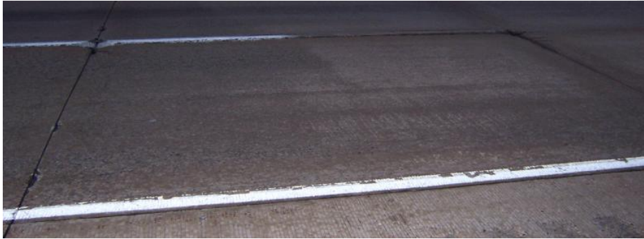
Figure 47: Overall View of Slab 5 SR 202 Segment 440 Northbound
