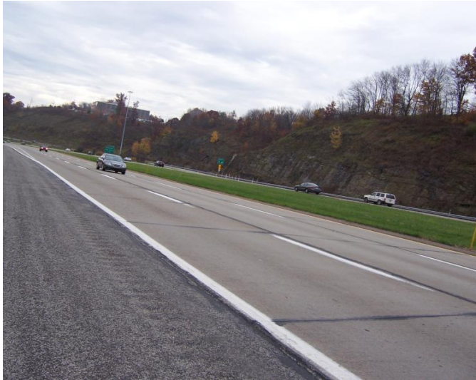
Figure 5: Overall Condition of SR 60 Segment 303 Southbound (Control Section).
