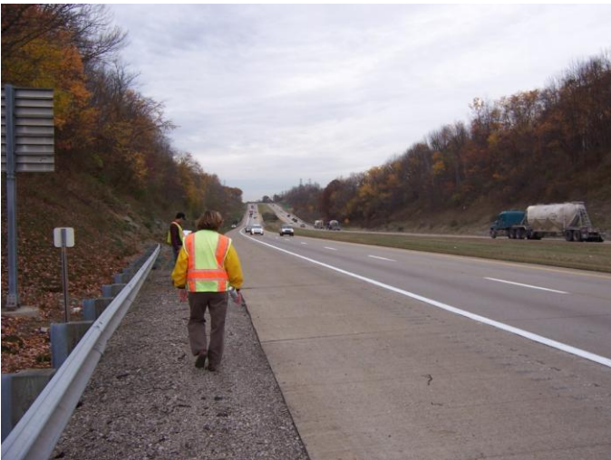
Figure 84: Overall Condition of I 79 Segment 480 Northbound (Control Section)
