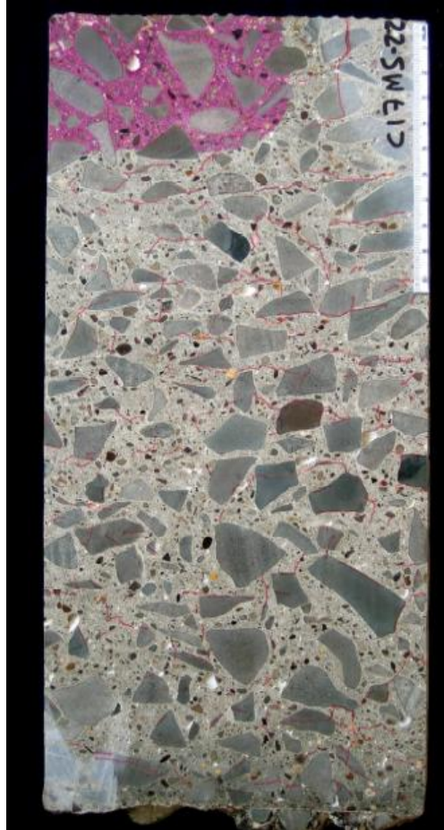
Figure 66: Development of ASR Gel in Carbonate (Coarse) Aggregate at Depth in Core C17-MS22 of US-22 Murrys ville, Westmoreland County Segment 50 Eastbound.
