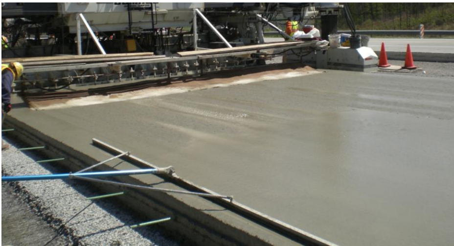
Figure 77: Wet Burlap Drag and Finishing Behind the Paver
