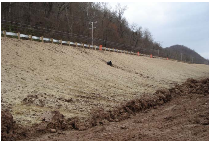
Figure 5.17: The Restored Embankment at WAS-7 Site.
