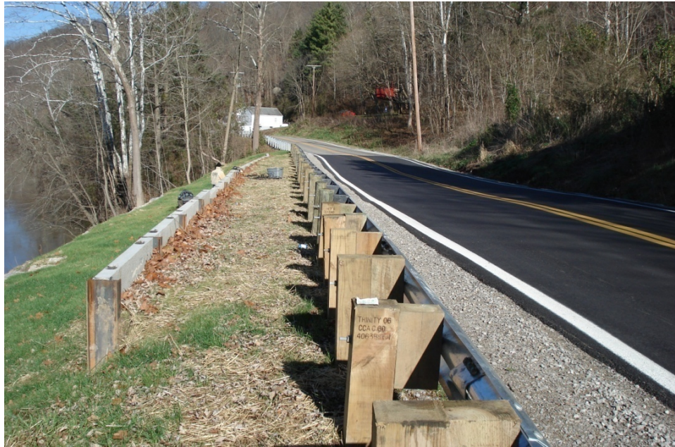
Figure 5.34: A Picture Showing the Restored Slope at MRG-376 Site
