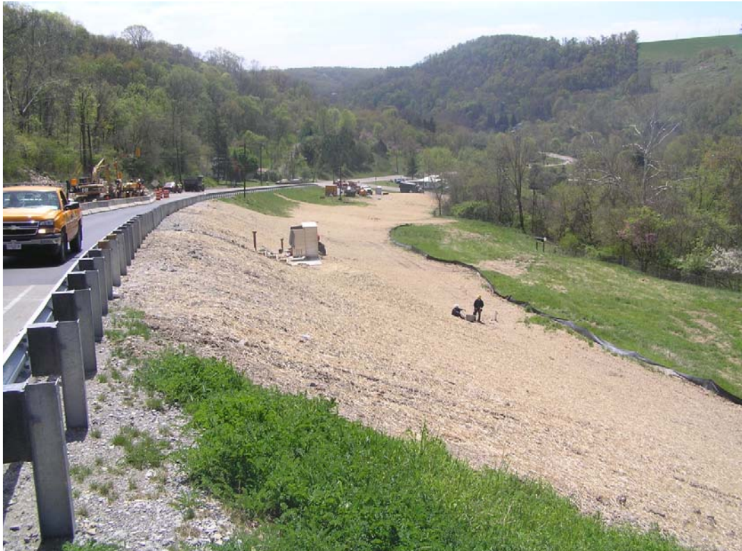
Figure 5.2: The Re-constructed JEF-152 West Embankment
