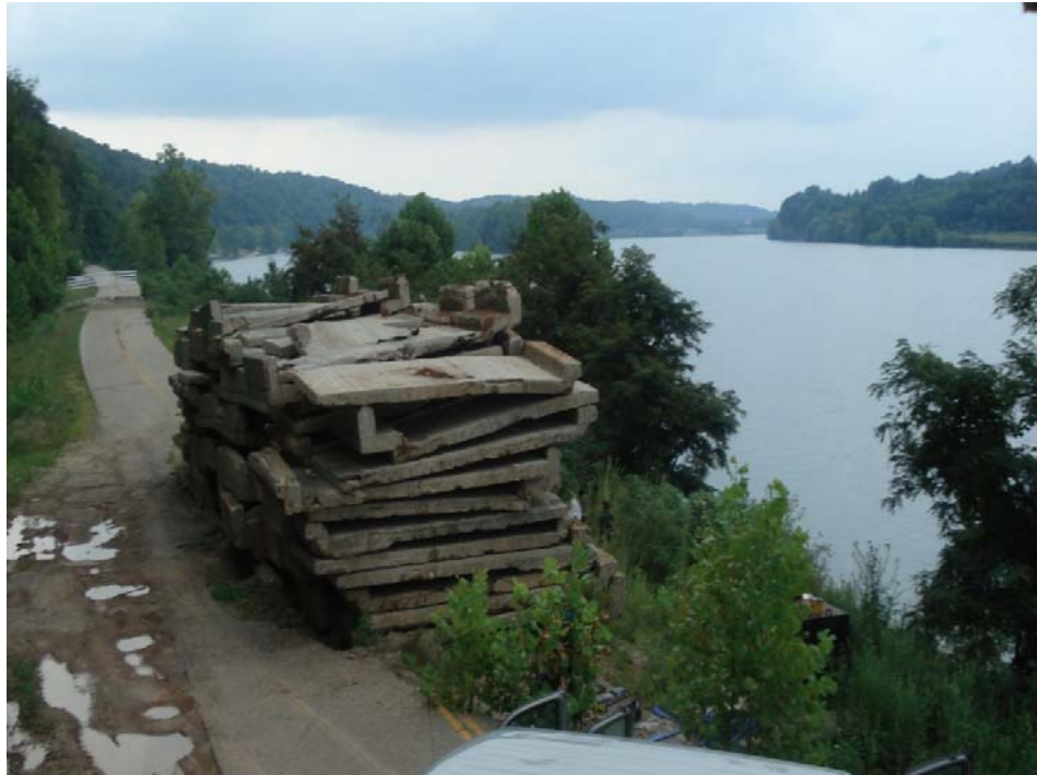
Figure 4.15: A Picture Showing the Surcharge Load Placed at the Test Site
