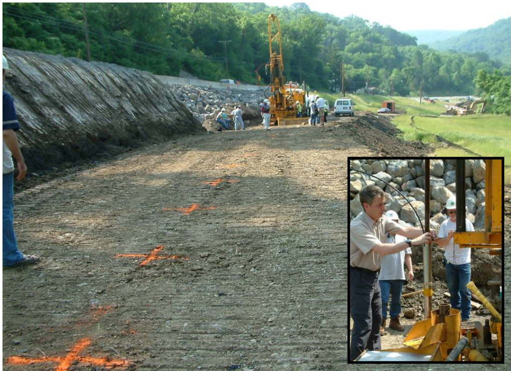
Figure 5.1: JEF-152 Failed Slope under Repair
