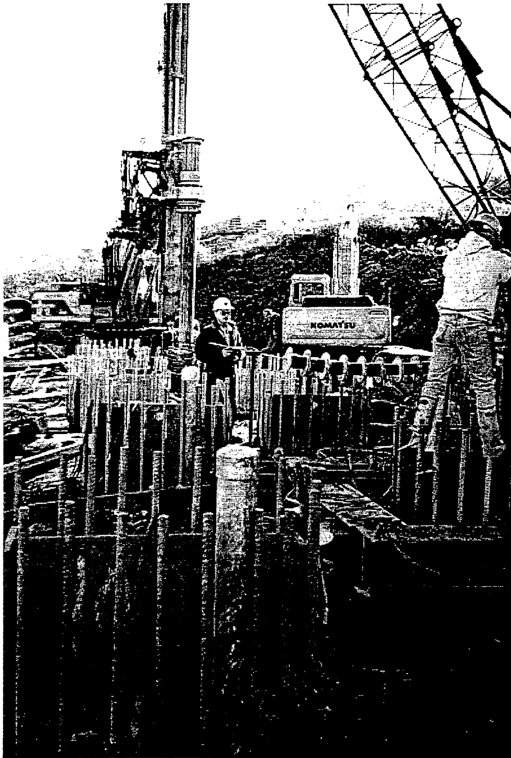
Fig. 7.15: Inclinator casing in drilled shafts.
