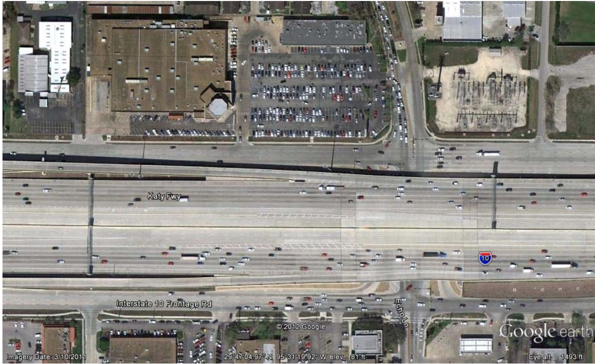
(a) Beginning of Cross-Facility Weaving Area at WB Access #6
