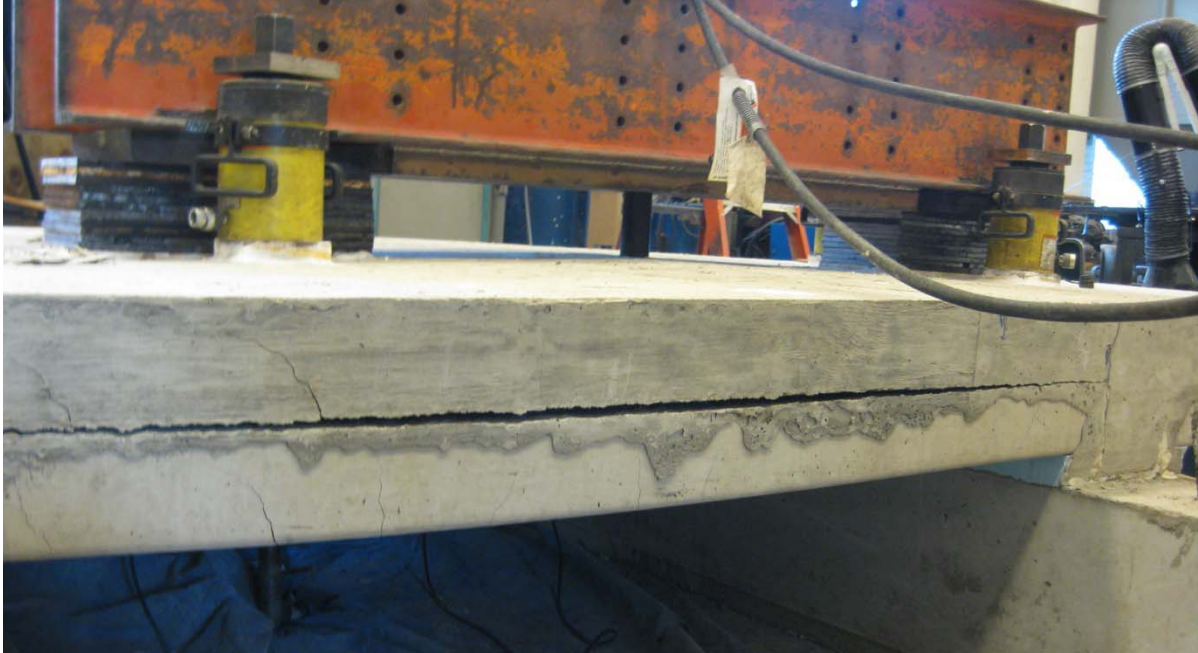
Figure 40: A sliding failure between the precast concrete panel and the cast in place concrete topping for Specimen B (standard TxDOT bridge deck). Note that this failure occurred at 8.7 times the design load.
