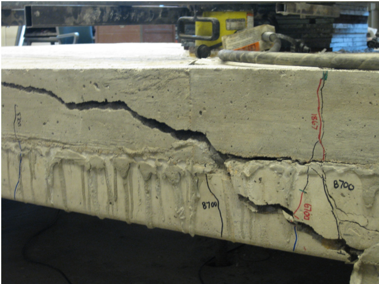
Figure 39: A punching shear failure of specimen A.
