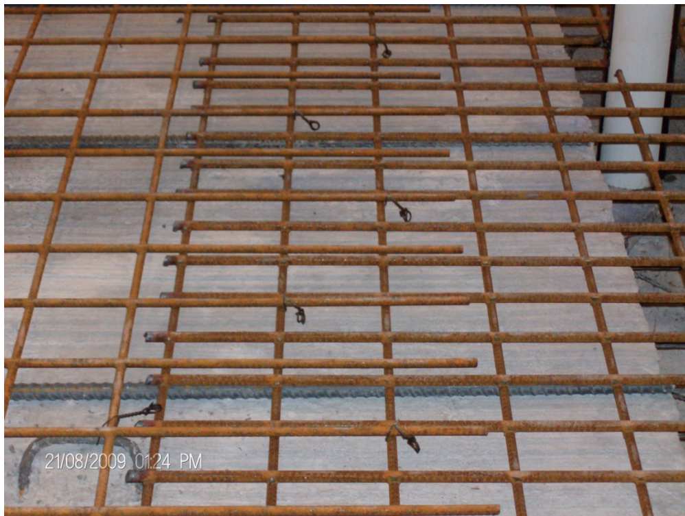
Figure 35: A splice between the two wire mats.
